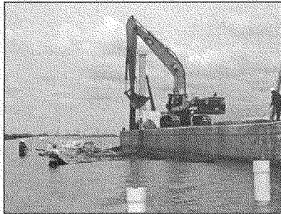
Placement of the bottom layer of geotextile fabric over existing foundation in native foundation displacement reach. (USACE)
