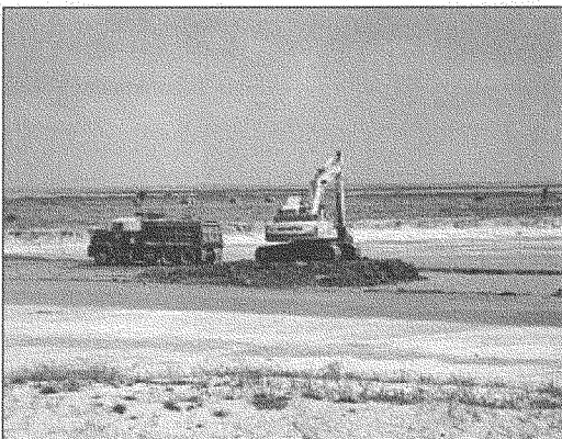
Heavy equipment operators remove excess material to create one of the channels connecting the three basins within the Bahia Grande wetland complex, Texas. (Tbor Lassen, Ocean Trust)
