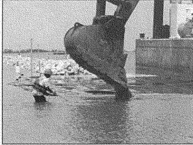
Placement of sand foundation on geotextile in native foundation displacement reach. (USACE)
