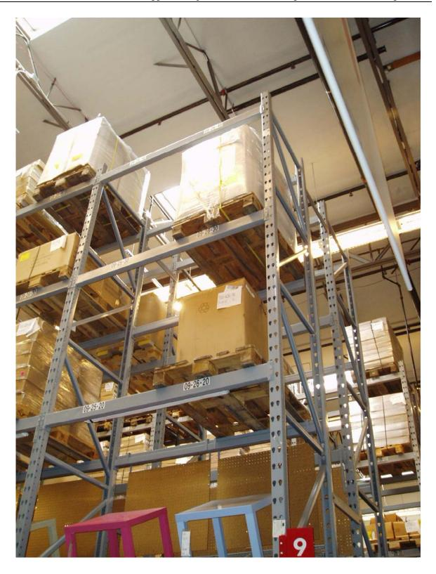
Figure 8-2 Pallets in this home furnishings store are supported only on the beams and may slide off these supports during an earthquake.
