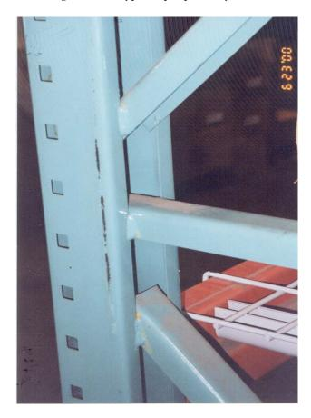
Figure 1-4 Typical rack bracing members and connections.
