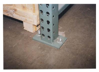
Figure 1-5 Typical column base plate connection.
