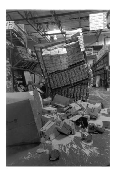
Figure 2-3 Cross-aisle collapse at Santa Clarita store showing good performance of shrink wrapped merchandise.
