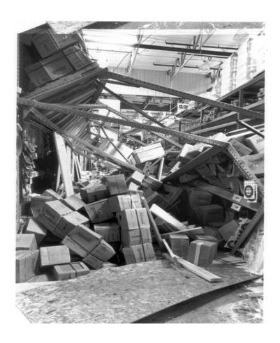
Figure 2-2 Cross-aisle collapse in the tile section of the Santa Clarita store.
