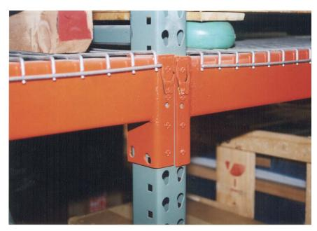
Figure 1-3 Typical proprietary moment connection.
