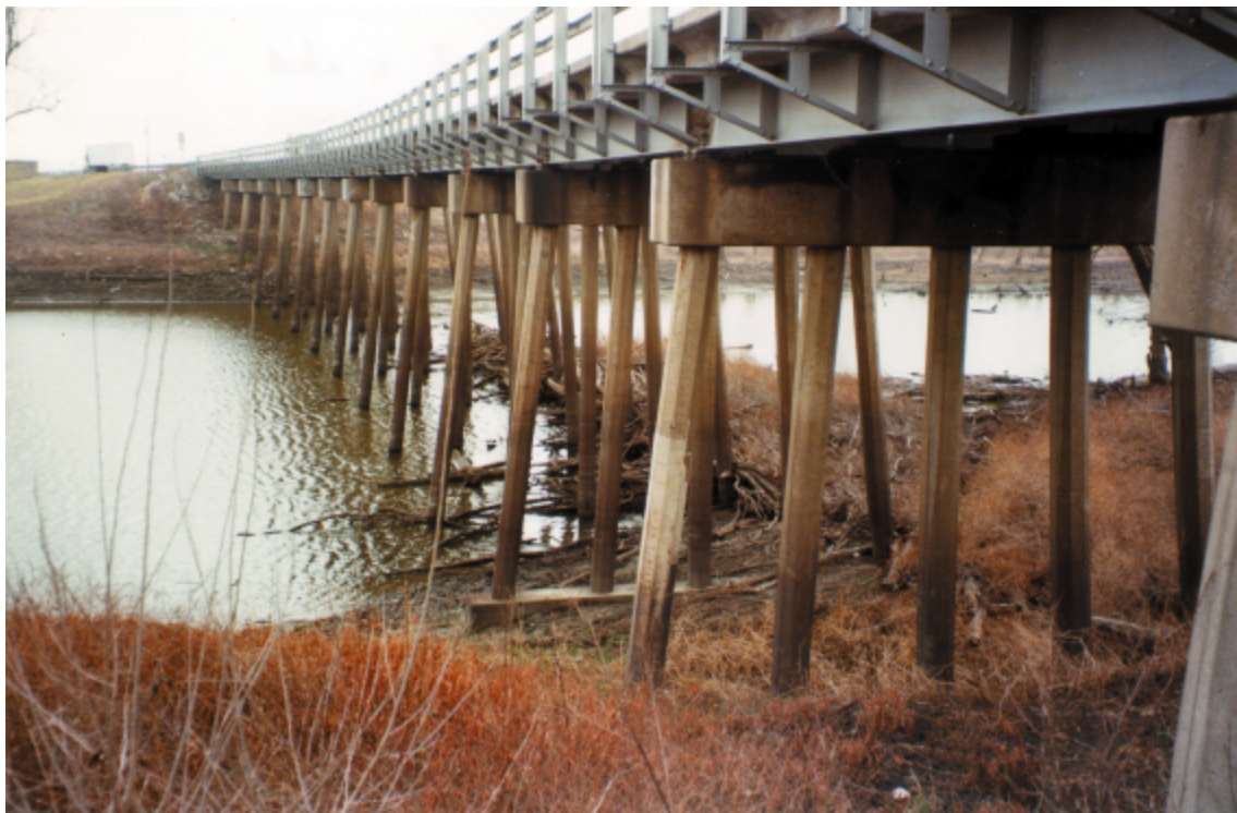
Figure 17. Downstream face of Horse Island Chute bridge near Chester, Illinois, as viewed from downstream face of left (north) embankment. Note debris trapped on upstream face of bents.
