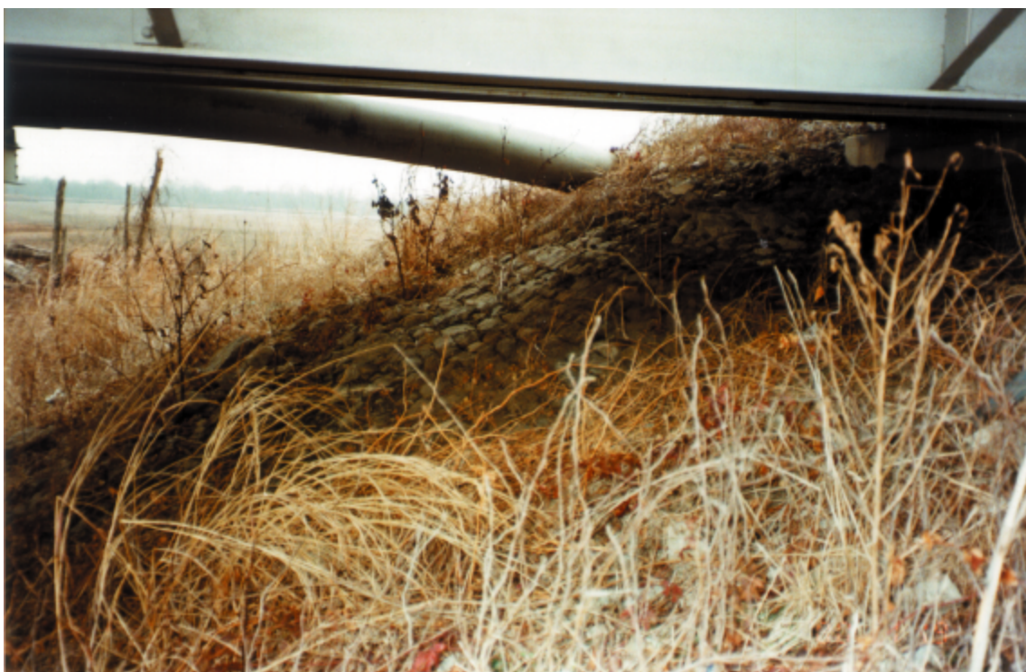
Figure 15. Stone revetment on abutment face under left (north) end of Horse Island Chute bridge near Chester, Illinois, as viewed from downstream face of bridge.
