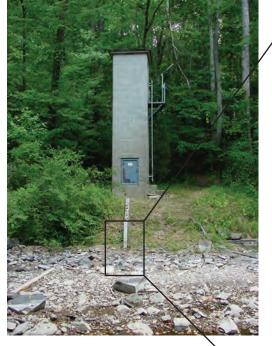
USGS streamgaging station at Big Bear Creek near Richfield (site 90, table 4), showing outside staff plate in dry streambed, June 19, 2002.
