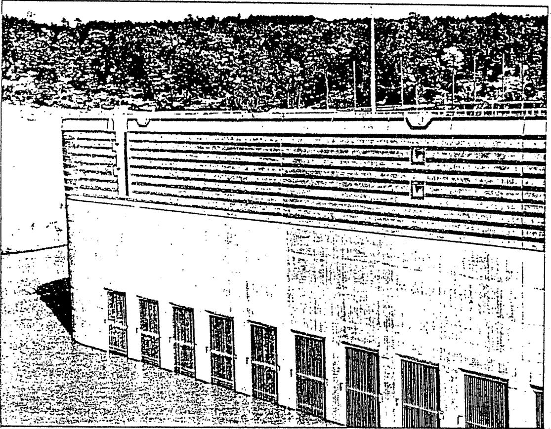
**Figure 8.23. Intake ports with trash racks in place during construction, Dardanelle Lock, Arkansas River.**
