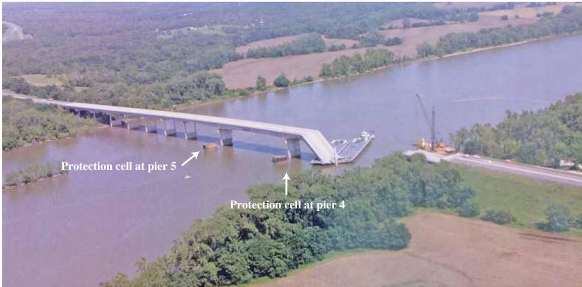
**Figure 14.** Upstream (northern) view of I-40 bridge showing pier protection cells at piers 4 and 5. (Source: ODOT)
