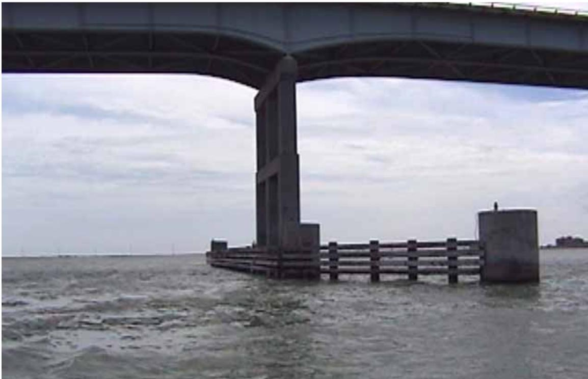
**Figure 18B.** Pier protection on east channel pier.
