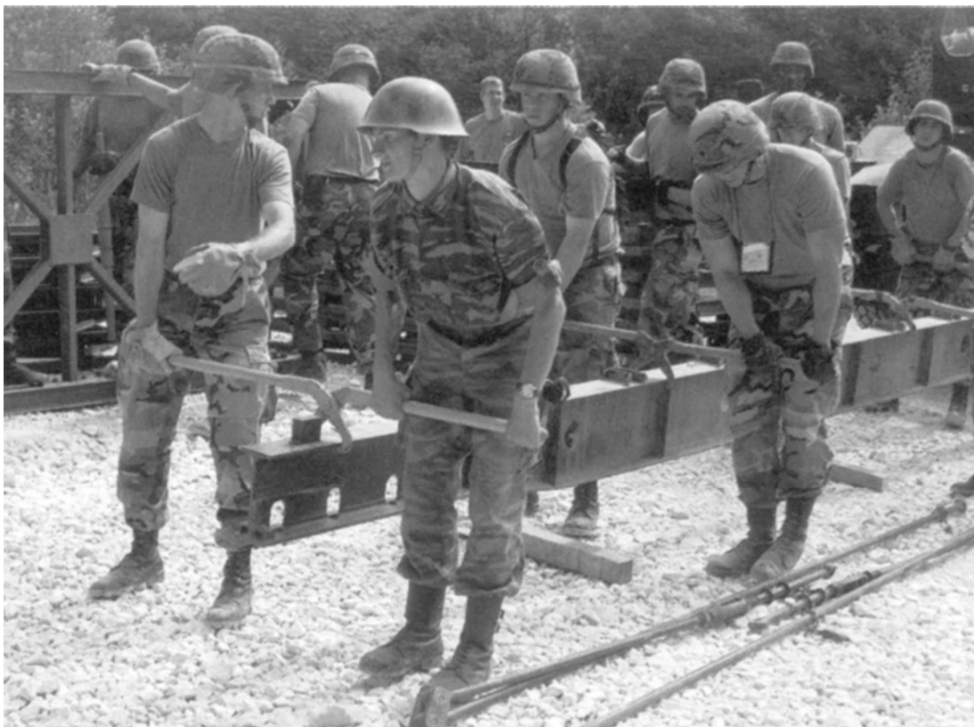
Members of the 43rd Combat Engineer Company work with engineers from the Srpska Entity Army to erect a Bailey bridge across the Lukavica River in Bosnia. The new bridge allowed local people to move building materials to repair homes that were destroyed in earlier fighting.
