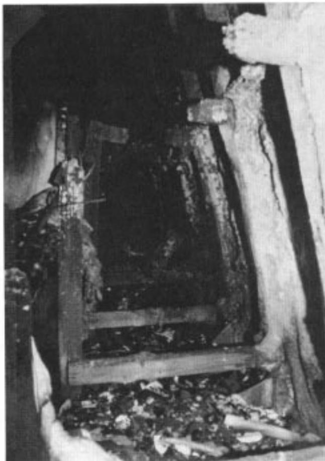
Figure 7 — Forward bulkhead of 02 deck. Shows construction details of wood framing over polyurethane foam insulation (courtesy NFPA, Quincy, Massachusetts)
