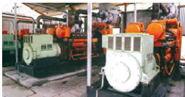
Electric generators operating on CMM: Jincheng Anthracite Mining Group, China.
