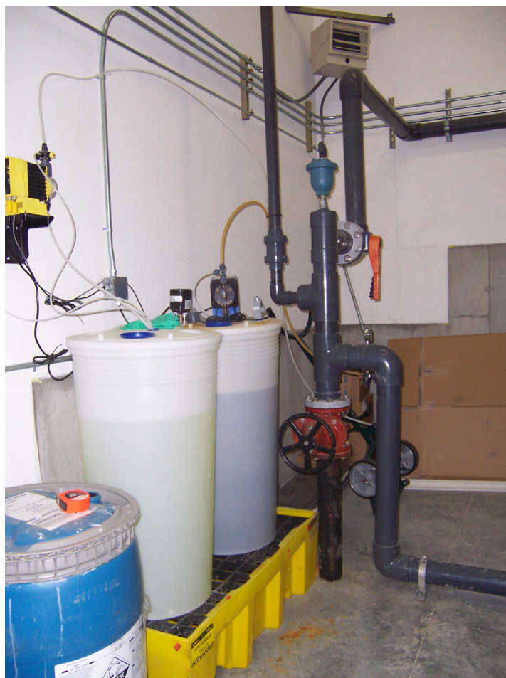
Figure 4-5. Chemical Feed Systems
