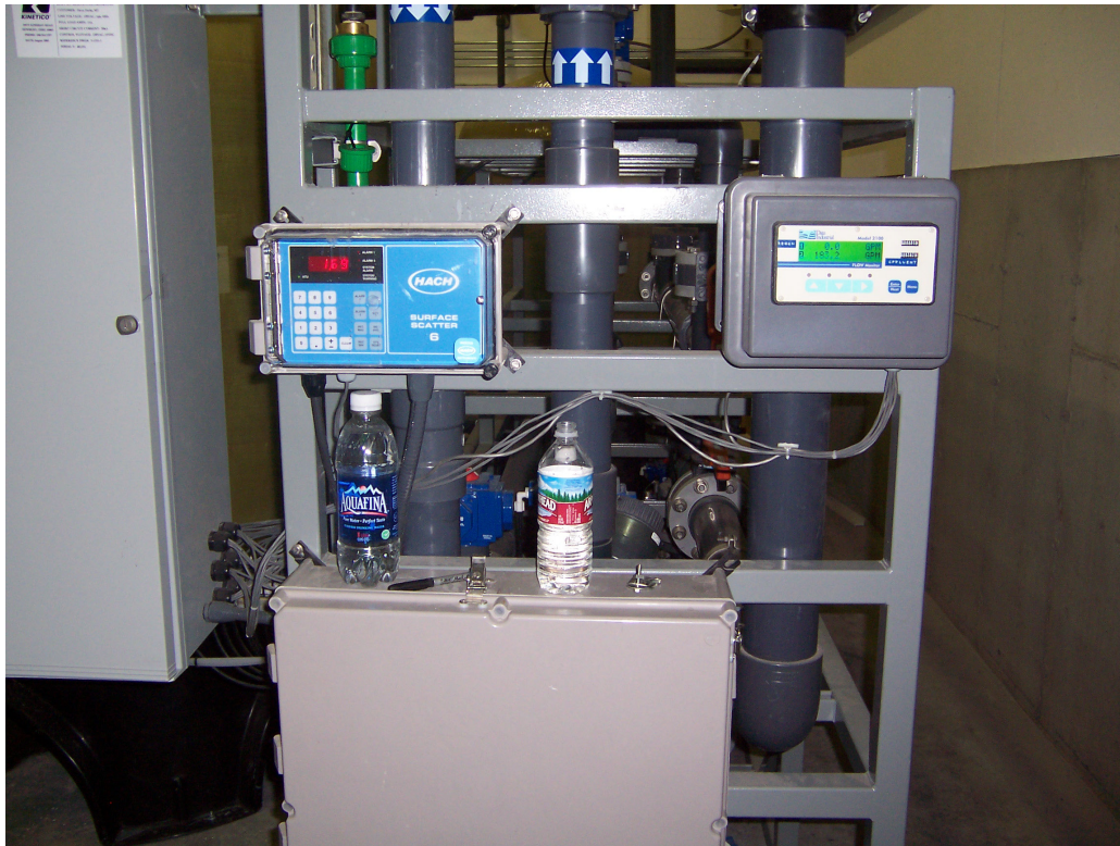
Figure 4-8. Hach ™ Turbidimeter for Control of Backwash Duration
