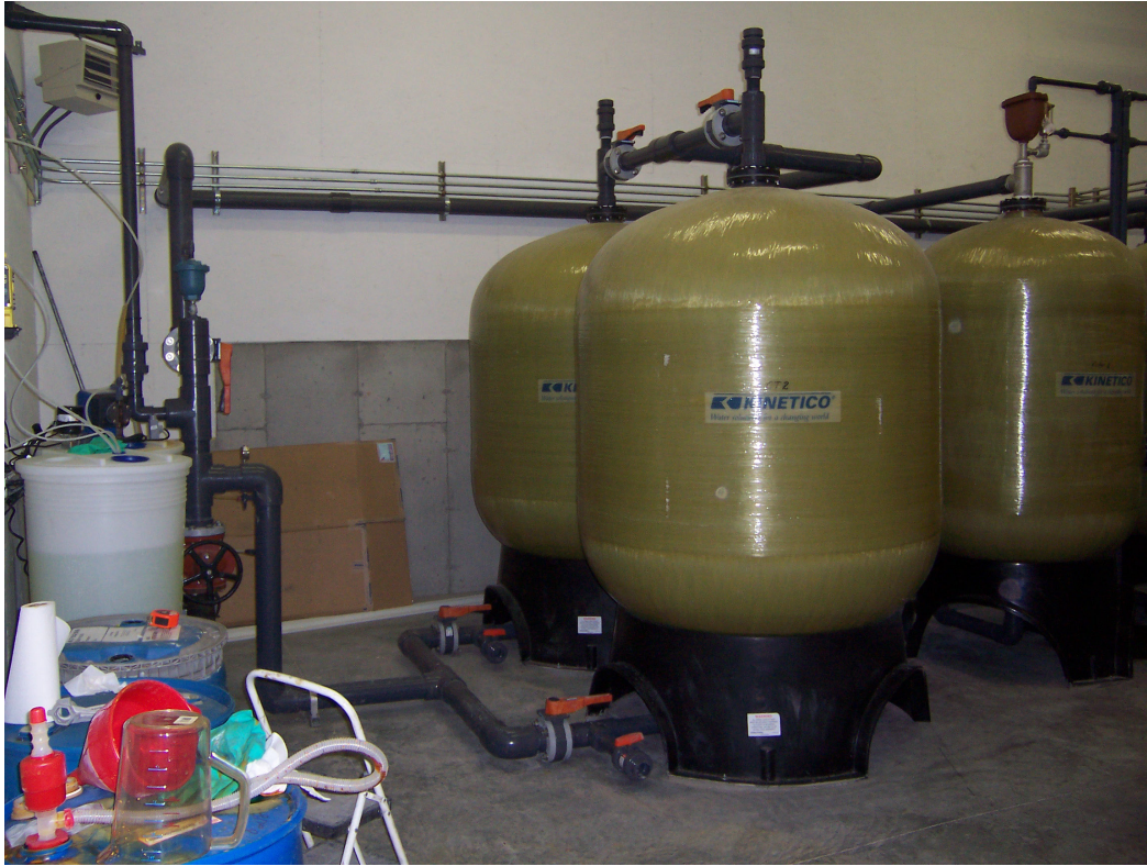
Figure 4-6. Contact Tanks with Inlet and Exit Piping
