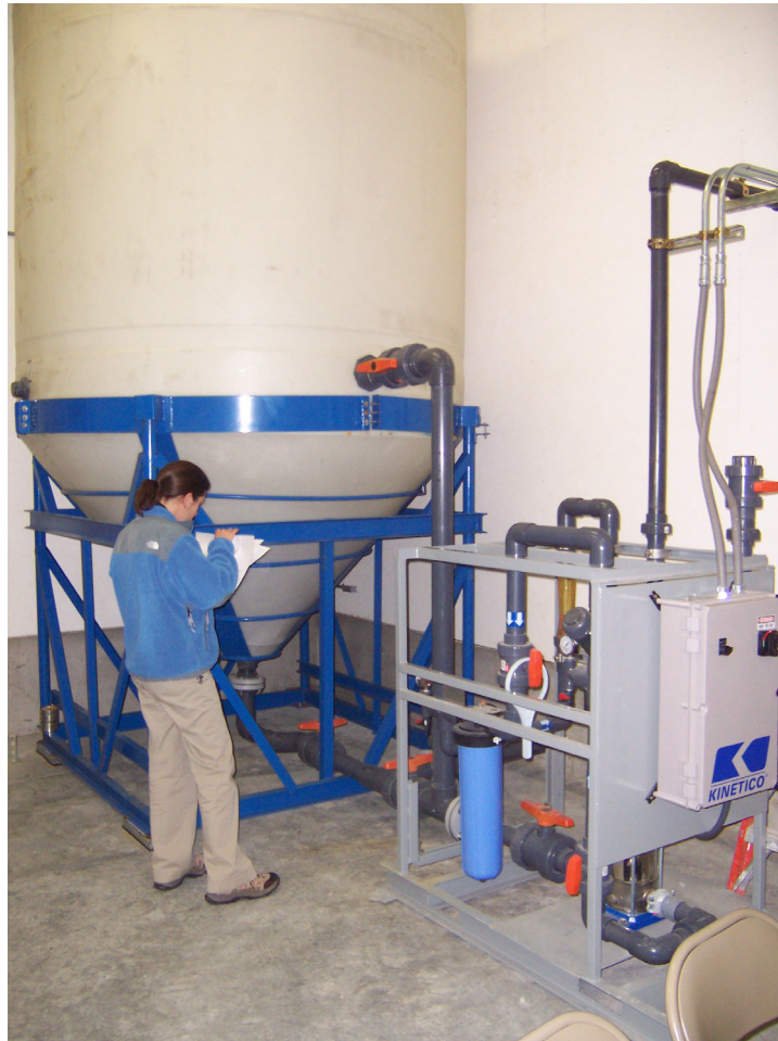
Figure 4-9. Backwash Recycle System
