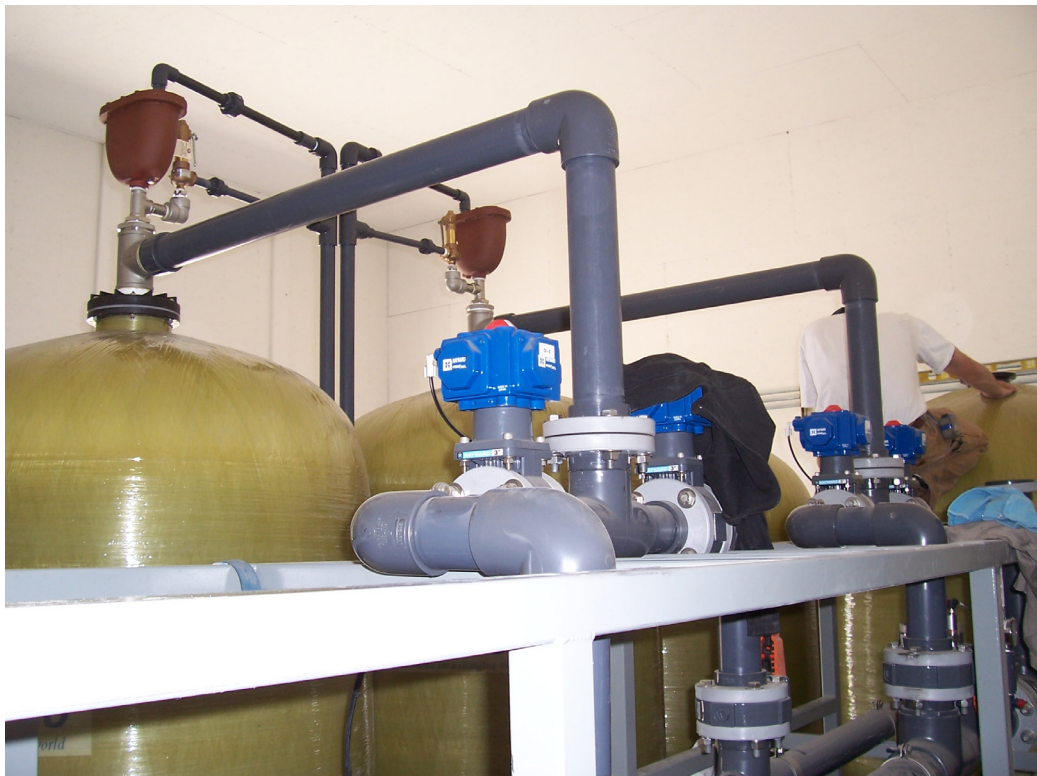
Figure 4-7. Filtration Vessels and Valve Rack
