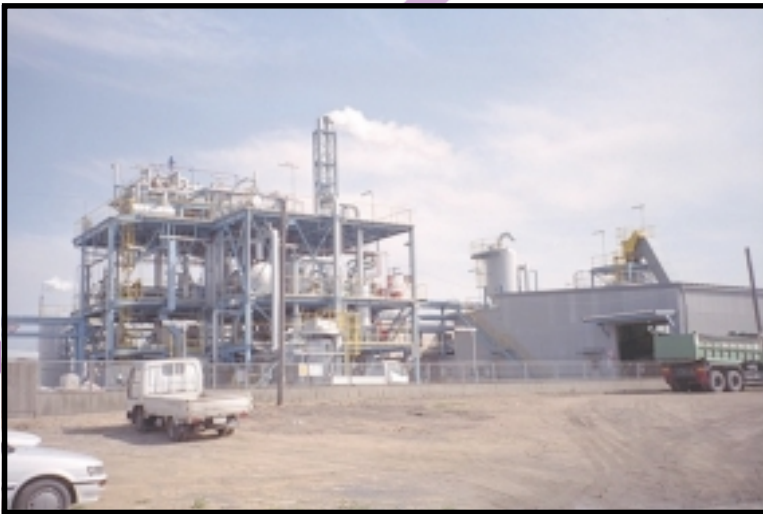
This 20 ton/day unit, which began operating in Japan in early March 1997, was designed as a fully integrated commercial-scale system for local MSW. The product fuel from the facility is cofired in a pressurized gasifier for hydrogen production or cofired in a cement kiln for heat production.
