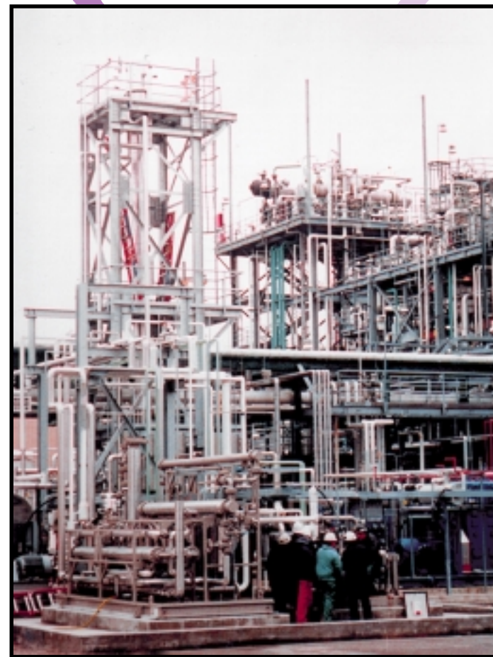
This MTR system was installed at a Huntsman Corporation Polypropylene Plant for recovery and direct recycle of propylene monomer.
