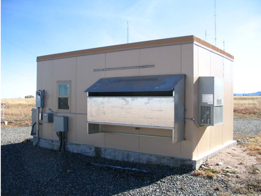
Figure 5. Diversion loads on exterior of data shed
