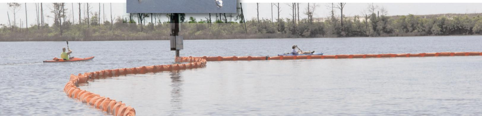
**Sorbent boom** looks like a long sausage. It is constructed of a long fabric sock enclosing material that attracts oil but repels water.
