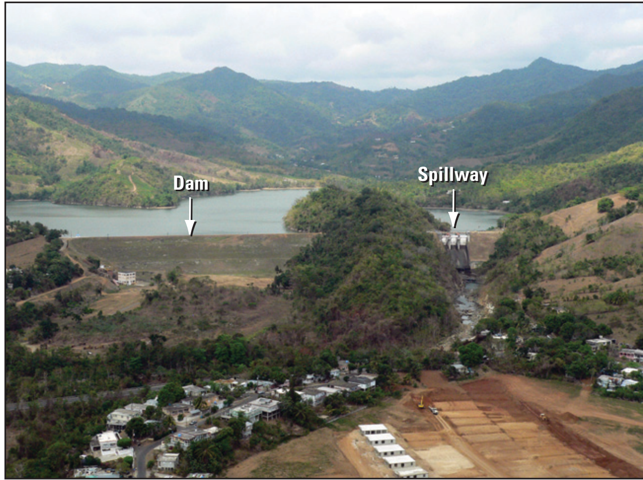
Figure 6. Aerial photograph of the Lago Patillas earthfill dam and spillway section. Photograph courtesy of the Puerto Rico Electric Power Authority.
