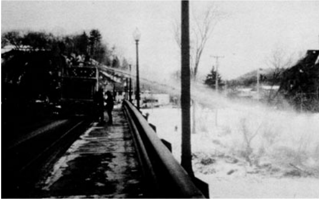
Figure 11. Hydroseeder being used to put leaves on the White River in Hartford, Vermont (March 1994).
