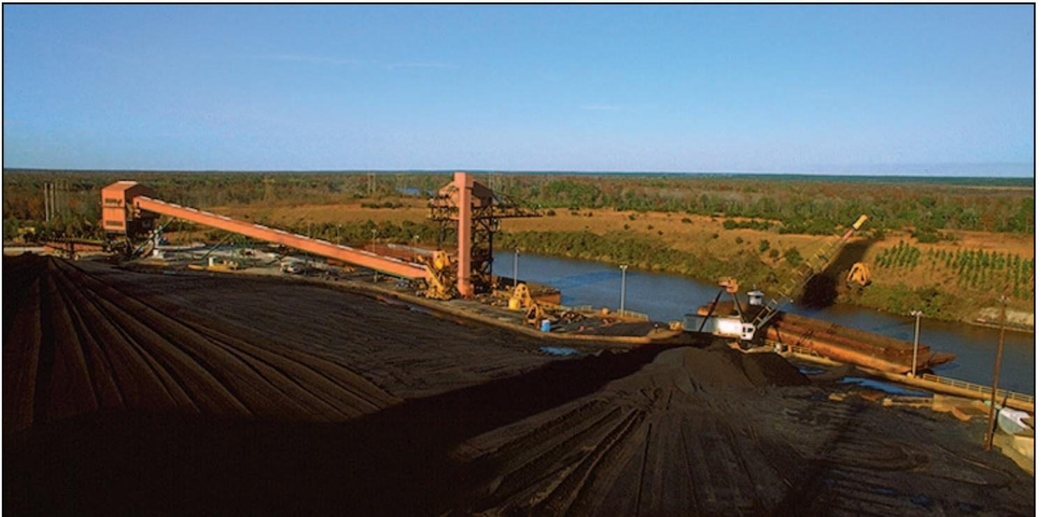
Coal barge unloading facility and storage area at Plant Crist
