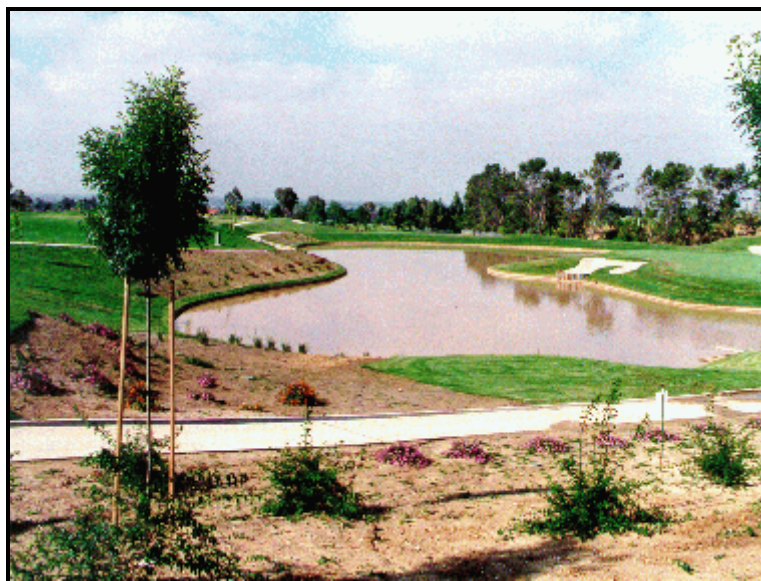
At the McColl Superfund site in Fullerton, California, designers included landscaped areas as part of a golf course built over a cover system. Designers omitted a layer of cobbles for covers over landscaped areas to minimize settlement caused by the weight of the cap, using institutional controls instead.
