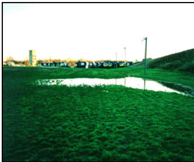
A soccer field built on a portion of the Fairfax County Municipal Landfill in Virginia illustrates the need to address settlement, which can cause depressions in the cap that can lead to drainage problems and poor field conditions.
