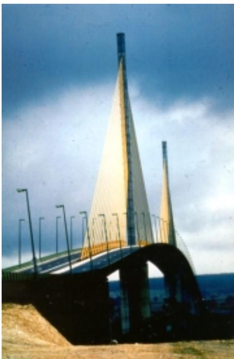
Figure 19. A detail built into the design enabled the cable stays of the Brotonne Bridge to be re-tensioned about 10 years after construction to adjust for long-term creep deformation.
