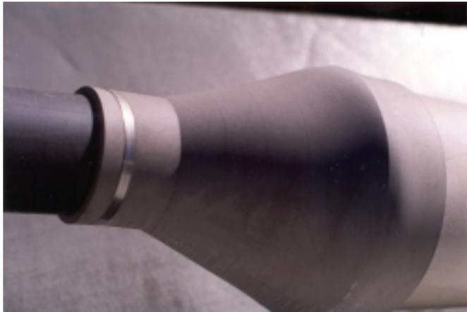
Figure 34. Cable-stay boot connects the external stay pipe to the transition pipe at the anchors on Sunniberg Bridge.
