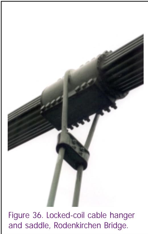
Figure 36. Locked-coil cable hanger and saddle, Rodenkirchen Bridge.
