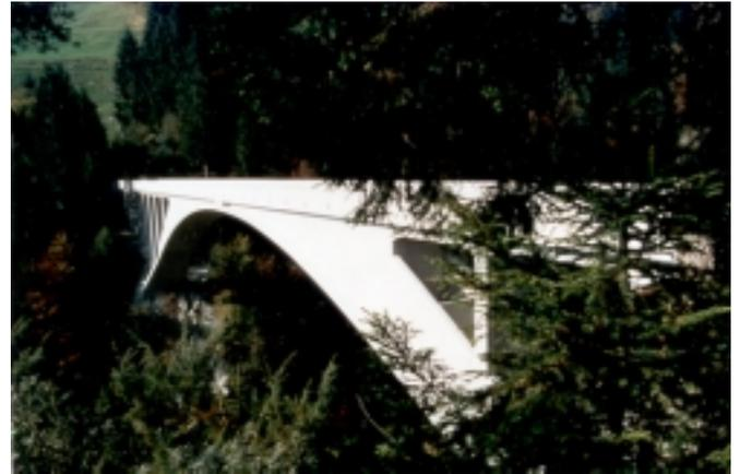
Figure 1. The Salginatobel Arch Bridge, with its reinforced concrete arch, was built in 1929 in Switzerland by Robert Maillart.
