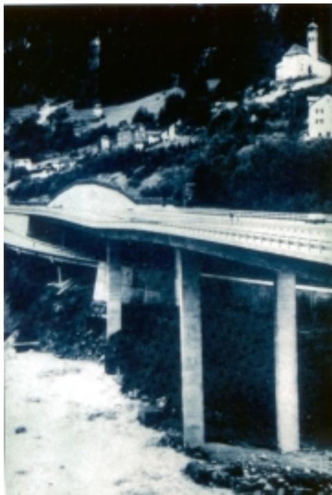
Figure 21. A main pier of the Reuss Bridge, at Wassen, was undermined by scour from excessive flash floods in 1987, but the bridge remained intact.
