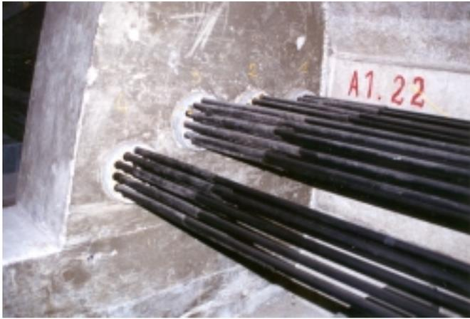
Figure 30. External, greased-and-sheathed mono-strand tendons pass through a diaphragm on Corbeil Bridge.
