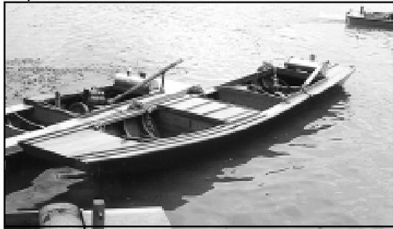
*The "putt-putt" was made by installing a two-cycle motor in a bateau or "joe boat."*
