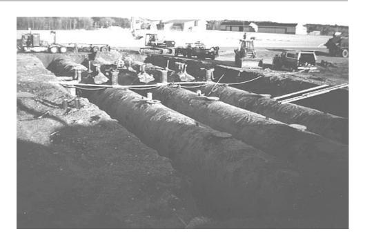
Figure 4: Underground Fuel Storage Tank Removal at Pease Air Force Base
