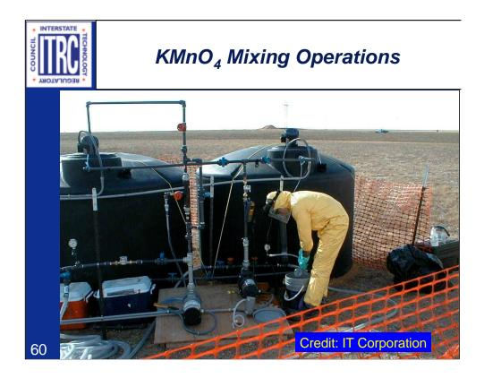
Batches of permanganate are mixed on site prior to injection.
