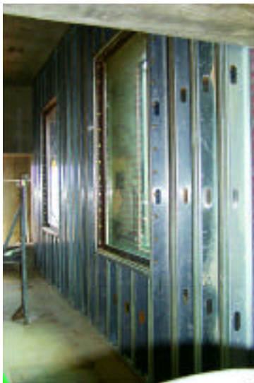
Figure 12. Pre-test Photos of Steel Stud Retrofit Walls Before and After Installation of Interior Gypsum Board.
