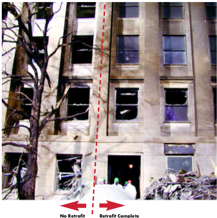
Figure 20. Window Damage from September 11 Attack on the Pentagon. The Aircraft Impact Area Was Approximately 135 ft. to the Right.
