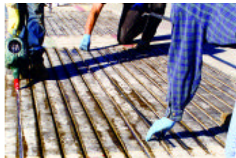
Figure 2. Placing Preformed Carbon Fiber Reinforced Polymer Rods Near the Top Surface.
