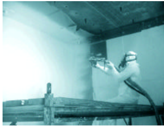
Figure 4. Application of Elastomeric Retrofit.
