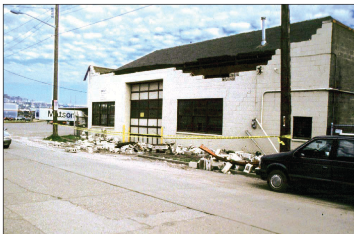
Figure 12. Partial collapse of URM building wall, Sodo neighborhood of Seattle.
