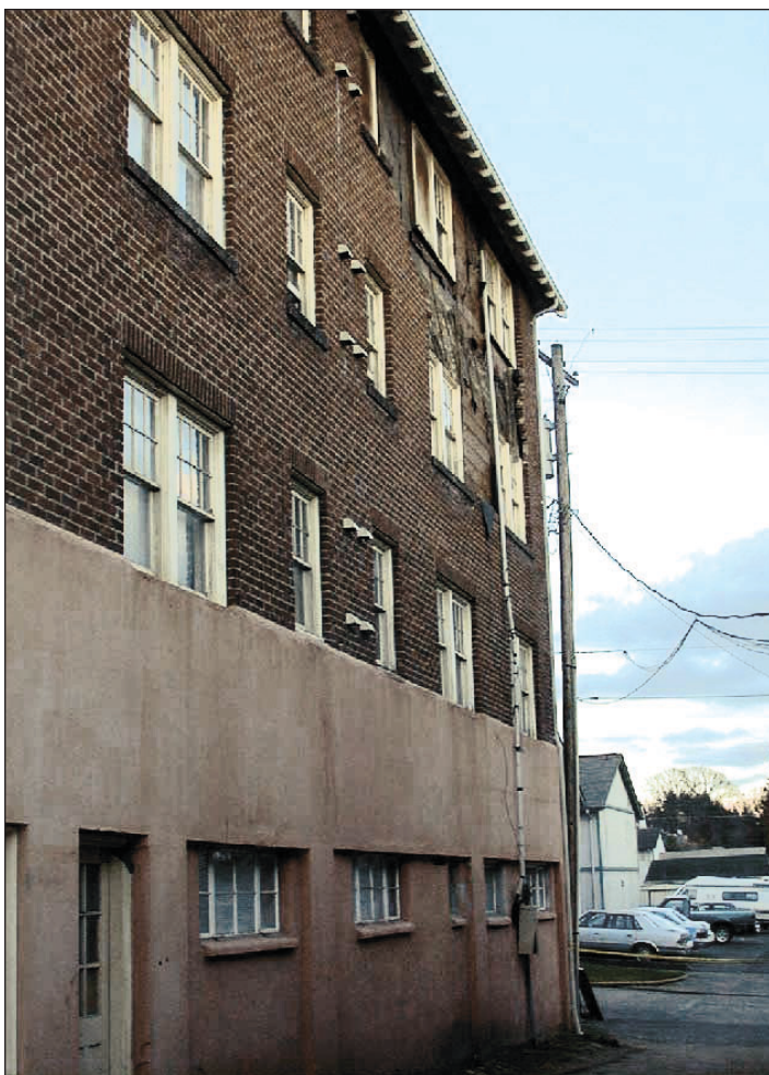
Figure 15. Brick veneer was peeled from the upper wall (near street) of this apartment building in Chehalis.
