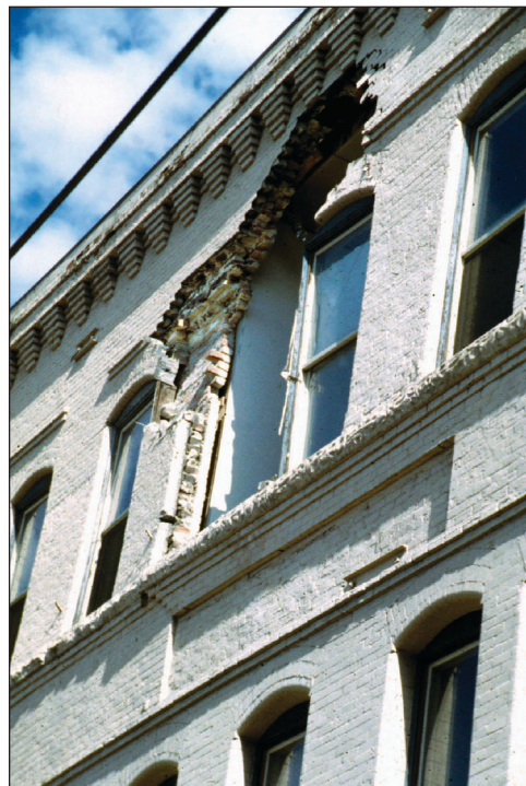
Figure 12. Partial collapse of URM building wall, Sodo neighborhood of Seattle.
