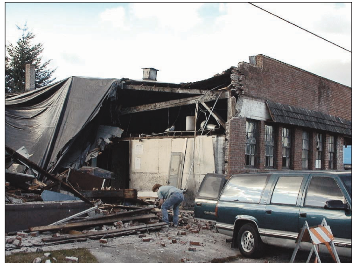
Figure 14. Unreinforced building in Centralia, damaged in the earthquake, and partially collapsed seven days after the earthquake.
