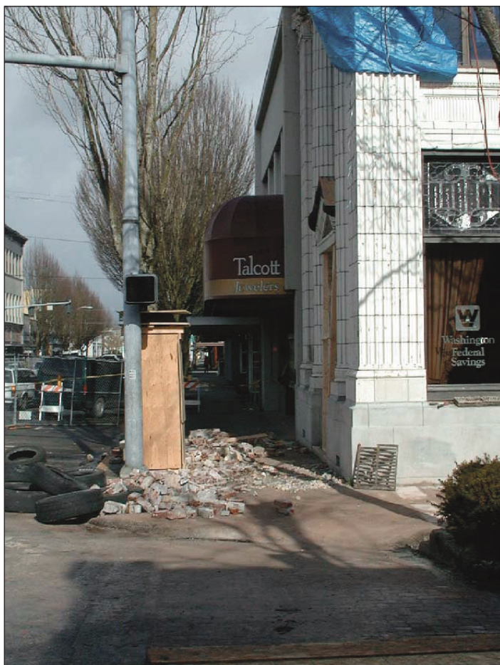
Figure 18. Bricks fallen from an unreinforced masonry parapet litter a sidewalk in downtown Olympia. In the Puget Sound earthquakes of 1949 and 1965, debris falling from buildings killed people on sidewalks below. Fortunately, this did not happen with the Nisqually earthquake.
