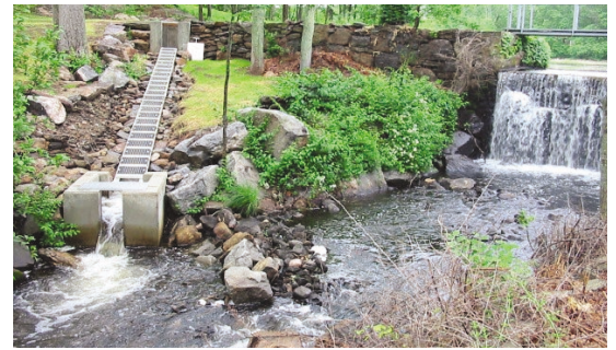
Newly installed fishway at the Upper Mill Pond Dam is part of a watershed-wide program to restore migratory fisheries to the Connecticut River. Photo: Courtesy of Chris Joyell, Connecticut River Watershed Council.
