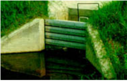
Outlet weir structures allow water level control for adjustment of hydraulic retention time.
