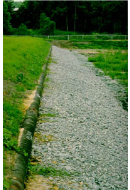
Influent distribution to the wetland cells is enhanced by perforated pipes on a rip-rap slope across the width of the wetland cells.
