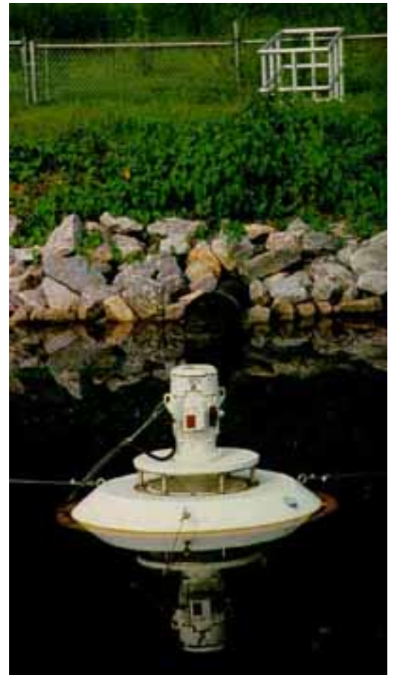
Post-aeration is essential for compliance with the effluent standard for dissolved oxygen.
