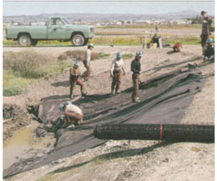
Biodegradable mesh was laid on banks near inlet and outlet structures during construction.
