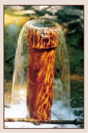
**Figure 5.** Depressurizing well flowing more than 100 gallons per minute near the MDA.
