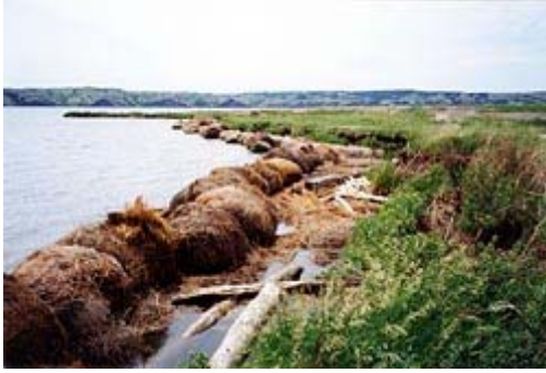
Figure 3. A farm where hay bales were put in place Sept/Oct of 1993. Note the height of the vertical cutbanks in the background, which are common to the entire lake. Lake Sharpe, South Dakota, June, 1994.
