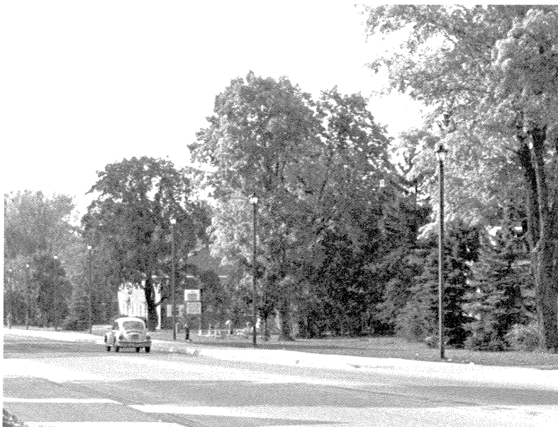
Figure 4.--Composite wood street lighting standards in Houghton, Michigan.
