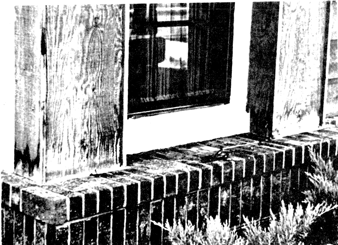
Figure 1.--Caulking incorrectly used instead of the recommended flashing.
