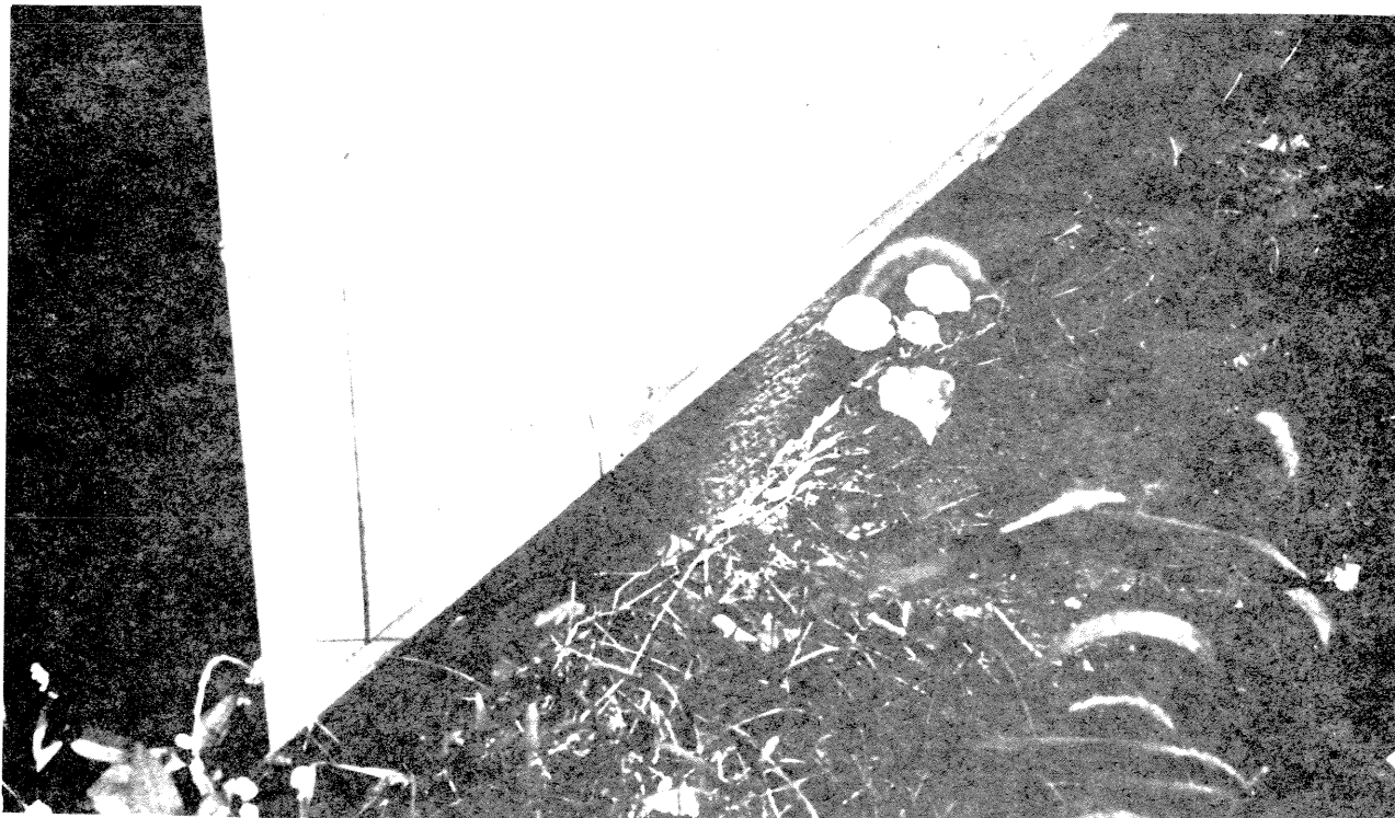
Figure 5.--The grade around the house improperly sloped.
