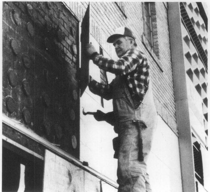
Fig. 16. A worker carefully removes a large glass panel by placing a small piece of wood between a flat prying bar and the glass, then exerting steady pressure. The majority of panels were removed without damage using this procedure. Photo: Thomas Keohan.
