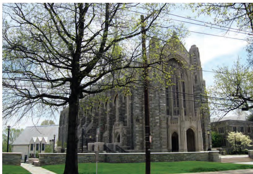
Figure 11. The addition to this early-20th century Gothic Revival-style church provides space for offices, a great hall for gatherings and an accessible entrance (left). The stucco finish, metal roof, narrow gables and the Gothic-arched entrance complement the architecture of the historic church. Placing the addition in back where the ground slopes away ensures that it is subordinate and minimizes its impact on the church (below).
