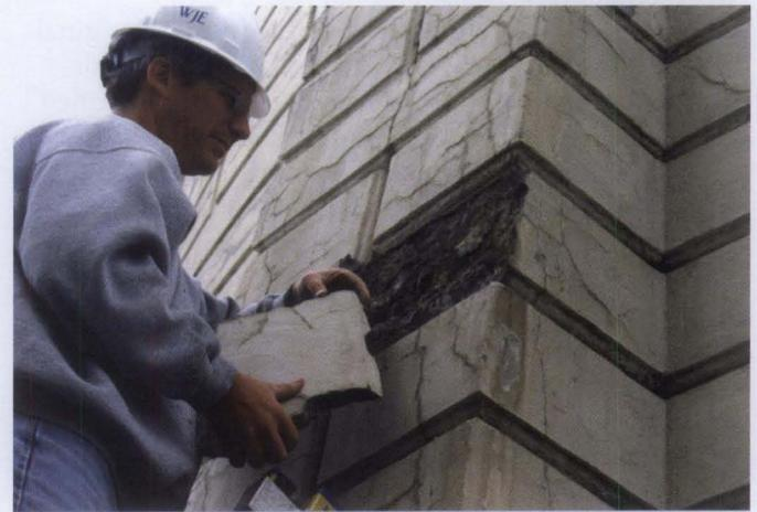
*Figures 14. Layers of architectural concrete that have debonded (spalled) from the surface were removed from a historic water tank during the investigation performed to assess existing conditions. Photos: Anita Washko, Wiss, Janney, Elstner Associates, Inc.*
