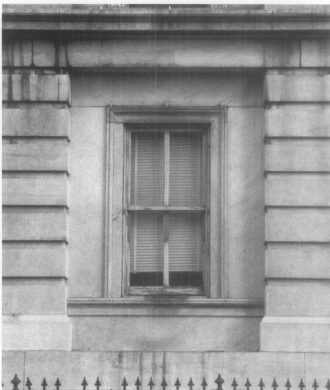
Fig. 10. Infiltration of damp air can occur around loose-fitting or deteriorated window sash and through cracks or open joints in building exteriors. Photo: Ann Brooks Prueher.
