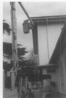
A. Inspecting the overall building on at least an annual basis will identify areas needing maintenance. A bucket lift is helpful for large buildings. Photo: author.
