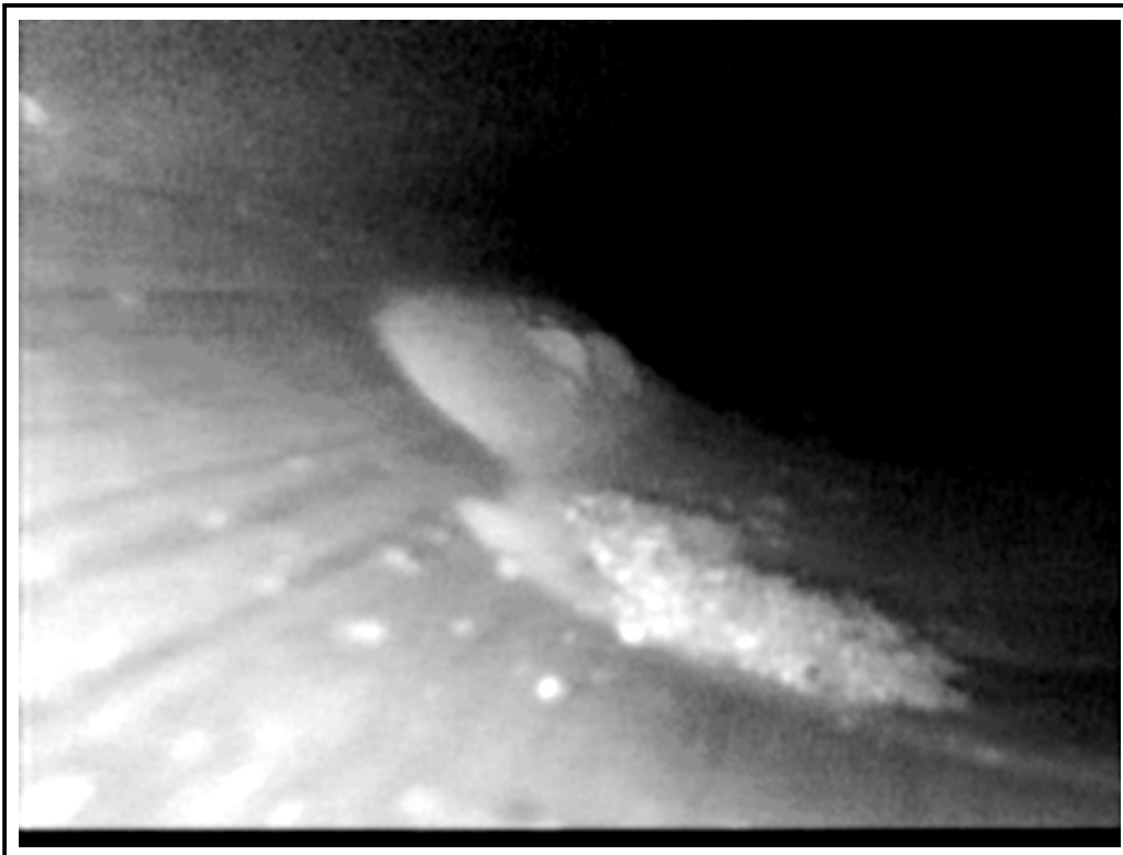
Figure 17. Silt resting on pipe bottom.
