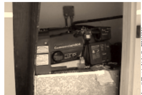
Propane generator compartment with installed exhaust housing
