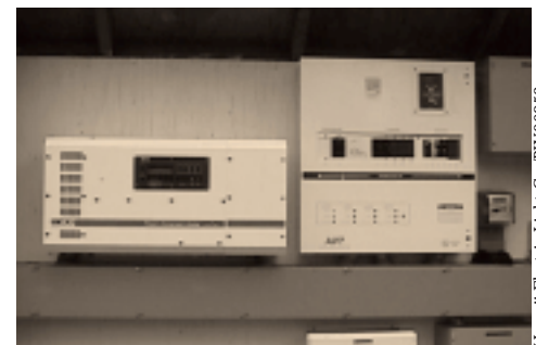
Inverter and charge controller
