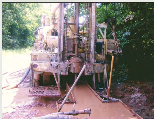
Figure 5. Drilling new, deeper residential well.
