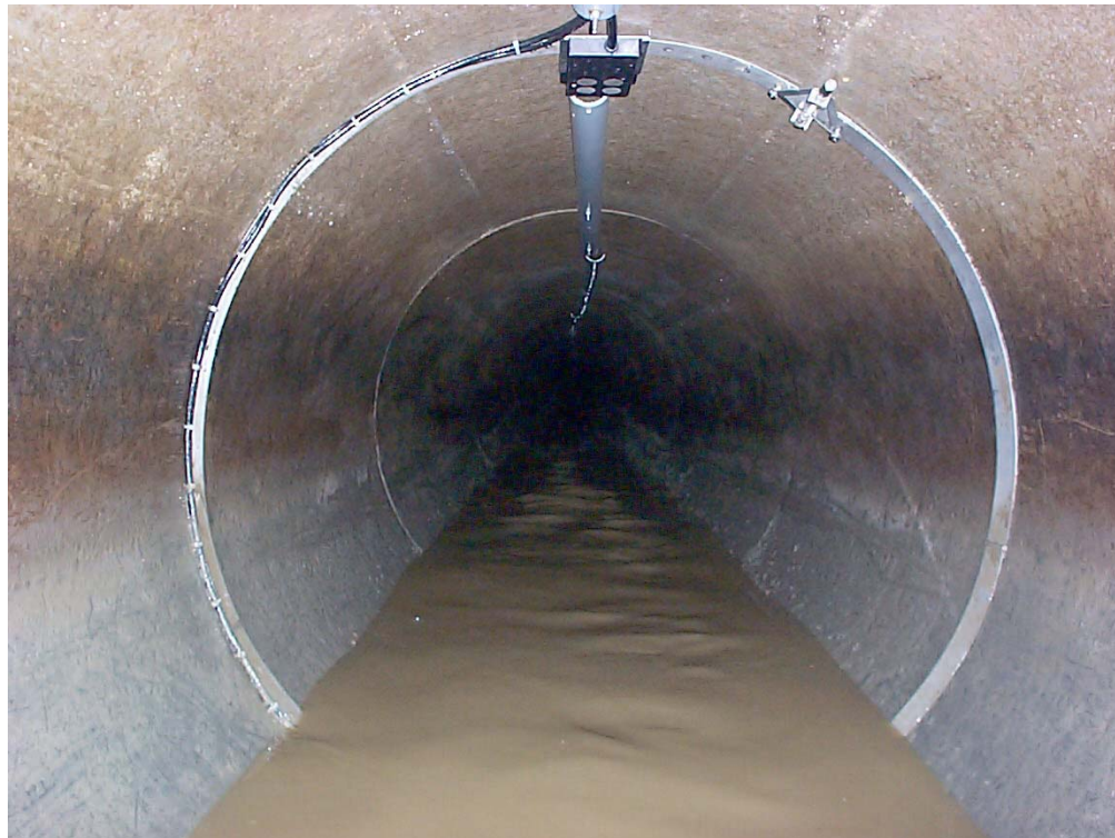
Figure 4-11. ADS 3600 flow meter installed in pipe.
