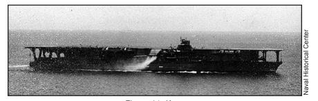
Figure 14. *Kaga*. Converted from a battle cruiser during construction. Completed in 1928; overhauled 1934-35. Displacement: 38,200 tons Maximum speed: 28 knots Crew: 2,016 Aircraft: 72 (90 in an emergency)
