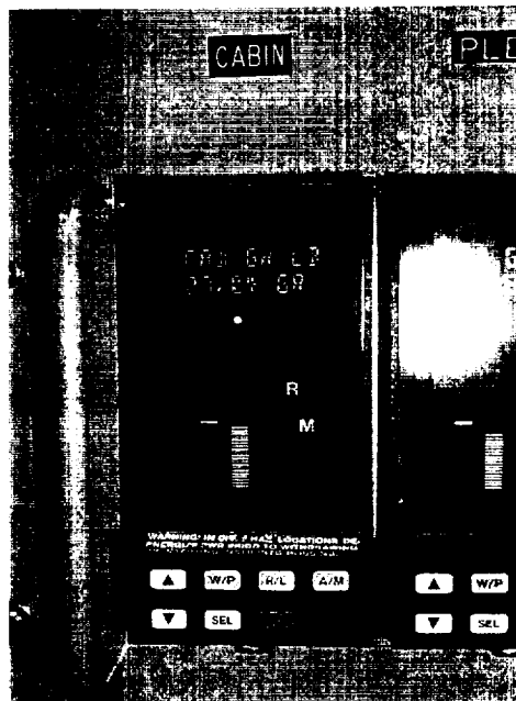
Humidifier Controller for the ECS at Pad 39-B
