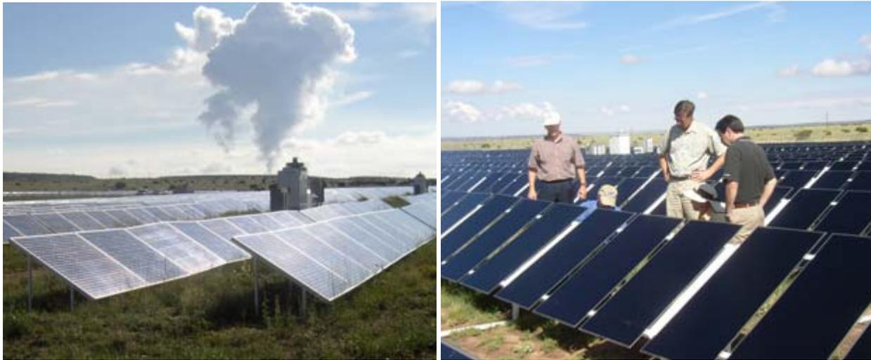
**Figure 1 PV sub-arrays at Tucson Electric Power in Springerville, AZ, made with 300 W (left) and 50 W (right) modules.**
