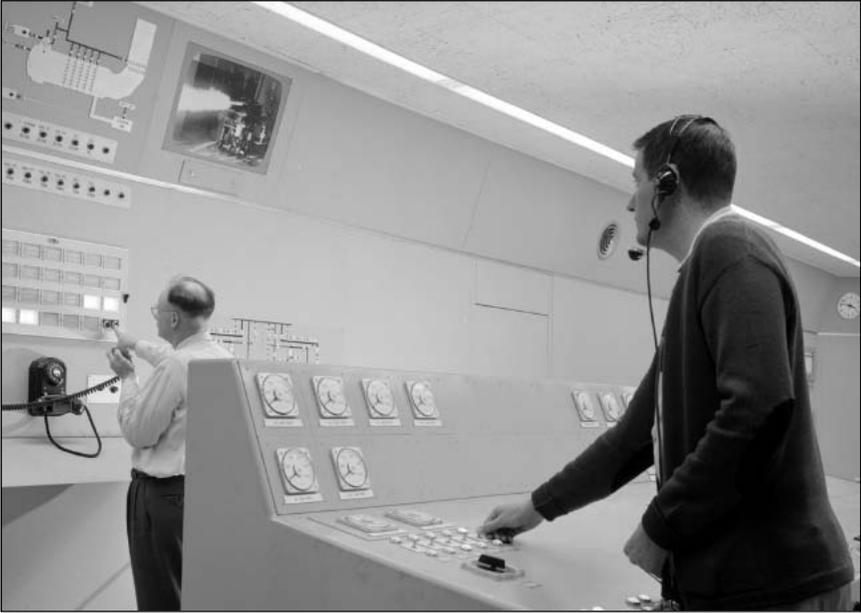
Operations engineers in the control room, located in Building 100, monitor early rocket tests, 1957. Video cameras in the test cell transmitted images during rocket firing. Instruments recorded pressures and other data that was later analyzed by the research engineers in charge of a particular test program.
