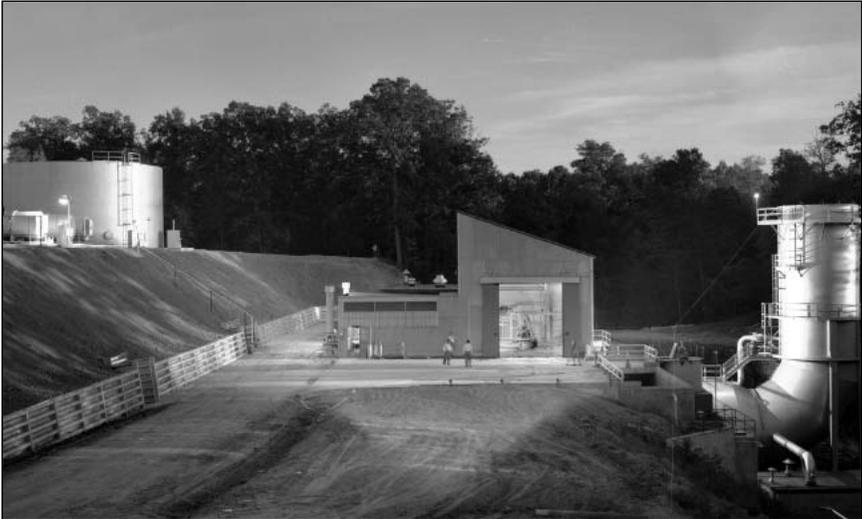
View of the test stand through the lighted open door of the test cell, also referred to as Building 202. The two men are standing on a cement apron where liquid hydrogen tanks would be installed in the spring of 1958. This photo appears to have been taken about the time of the NACA Triennial Inspection in October 1957.
