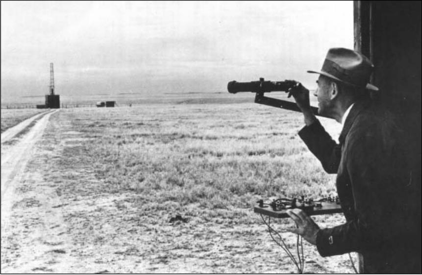
From a safe distance, rocket pioneer Robert Goddard uses a telescope to observe a rocket mounted in a test stand. His left hand rests on the control panel with keys for firing, releasing, and stopping a rocket test, undated, probably the 1930s.
