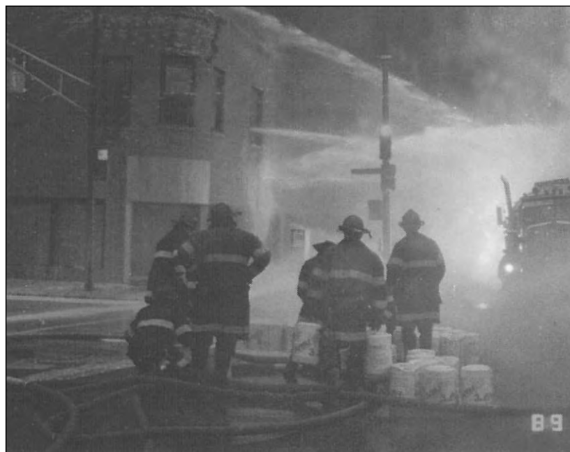
4. Firefighters operate foam handline to control spill fire. Note streams directed at exposure and tanker, including from second floor of exposure.
