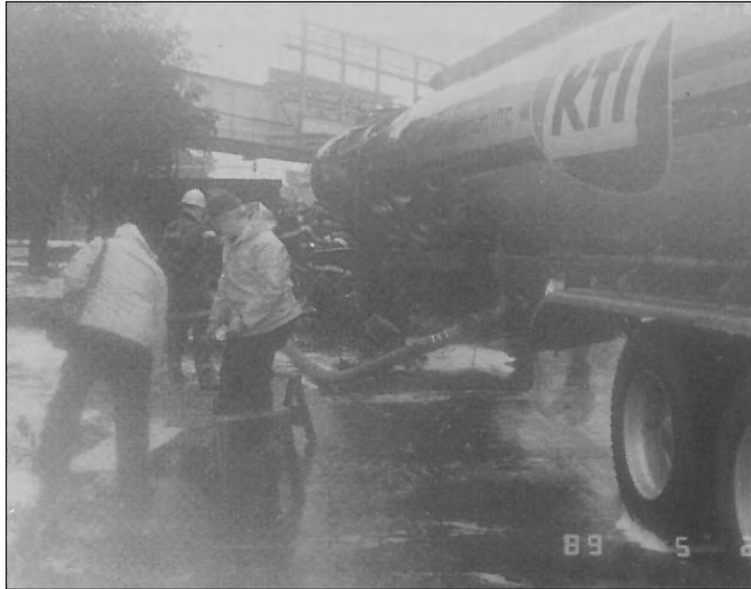
15. Off-loading in progress, water department employees check manhole for explosive vapors.
