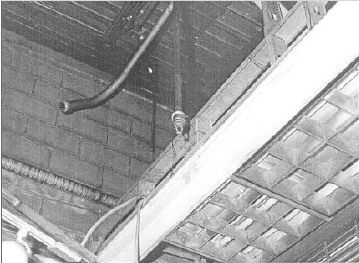
Photo 5. Open sprinkler head inside the store in Photograph 4. The ceiling tiles and grid around the head were removed before the picture. Typical concrete block tenant separation wall and metal deck roof construction in the older section. Interior tenant construction has used wood studs for the metal ones.
