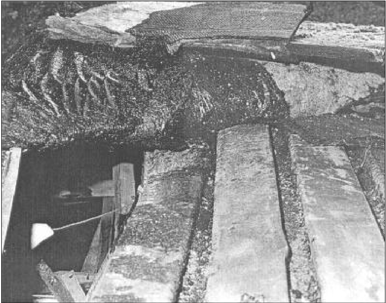
Photo 9. The top of the metal deck roof illustrating the insulation board, the vapor barrier under the board, the seam in the deck and the deformed condition of the metal. This section is in the partial roof collapse area shown in previous photographs.
