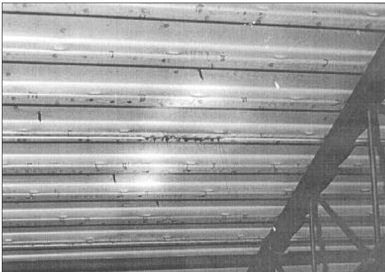
Photo 10. The underside of the metal deck roof above one of the stores adjacent to the covered mall. Note the tar dripping through the seam in the valley between metal deck sections. You can also see three mechanical fasteners poking through ridges in the deck. Such fasteners are usually found when less combustible roofing methods are employed.
