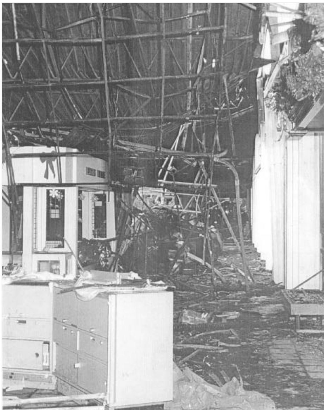
Photo 6. Moving further east in the covered mall, the counters in the foreground are also in Photograph 3. This area is where the metal roof began a partial collapse. The goods in the kiosks were either stored before the fire or removed prior to the picture.
