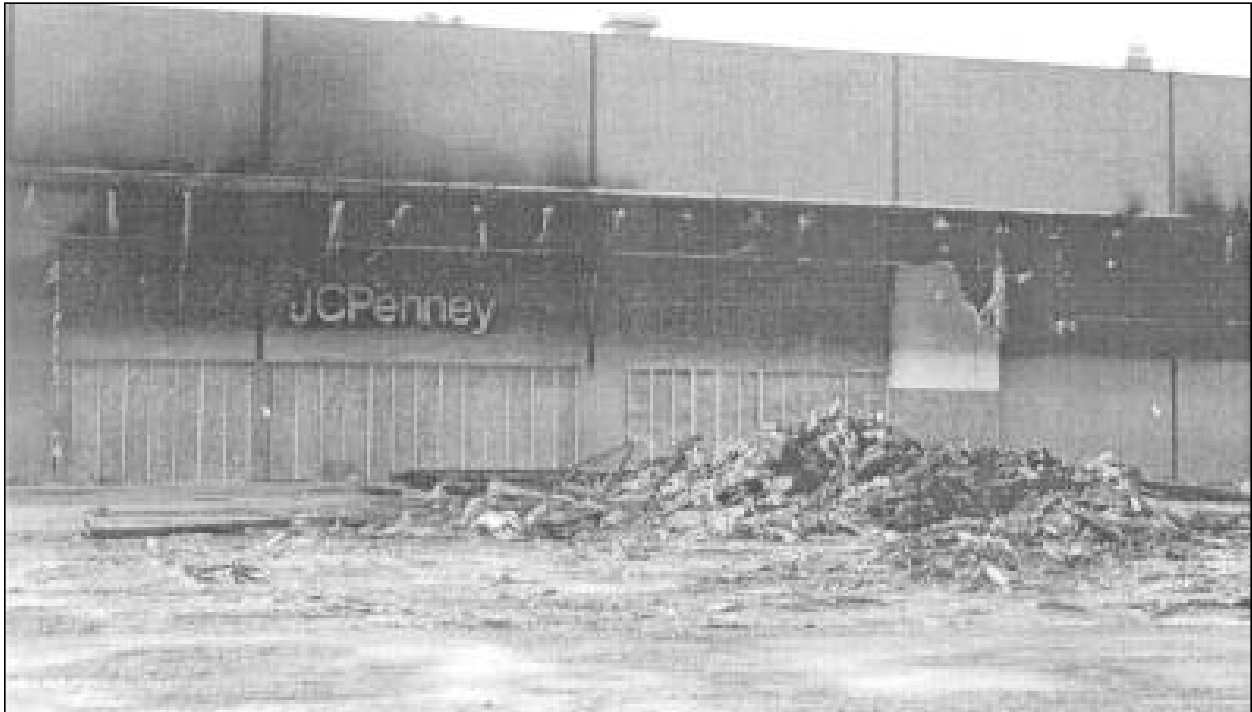
Photo 1. East wall of the J. C. Penney Store where the westerly fire travel was stopped. Roof line of covered mall is identified by the dark black horizontal line. Glass entrance and show windows are behind the chipboard and wood studs.
