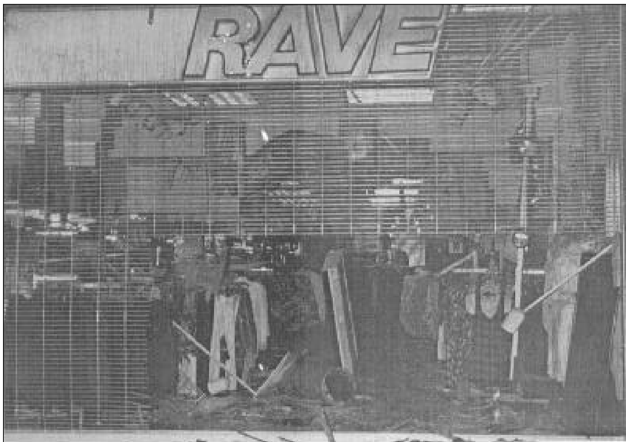
Photo 4. Store on the south side of the covered mall. Typical of the forcible entry work performed on the security grill and the damage to goods. This store had automatic sprinklers and the sprinkler heads at the front entrance operated.
