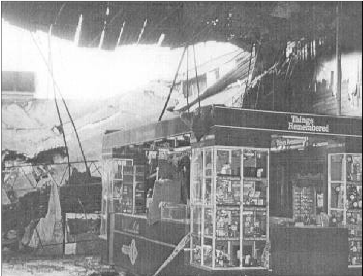
Photo 8. A front view of the partial roof collapse over the Things Remembered kiosk.
