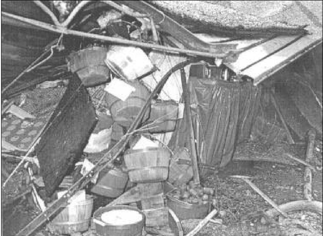
Photo 7. A candle kiosk under the roof collapse area shown in Photograph 6. Note that the candles, wicker baskets and table skirting are not melted or burned. Yet, the metal bar joist is severely deformed.
