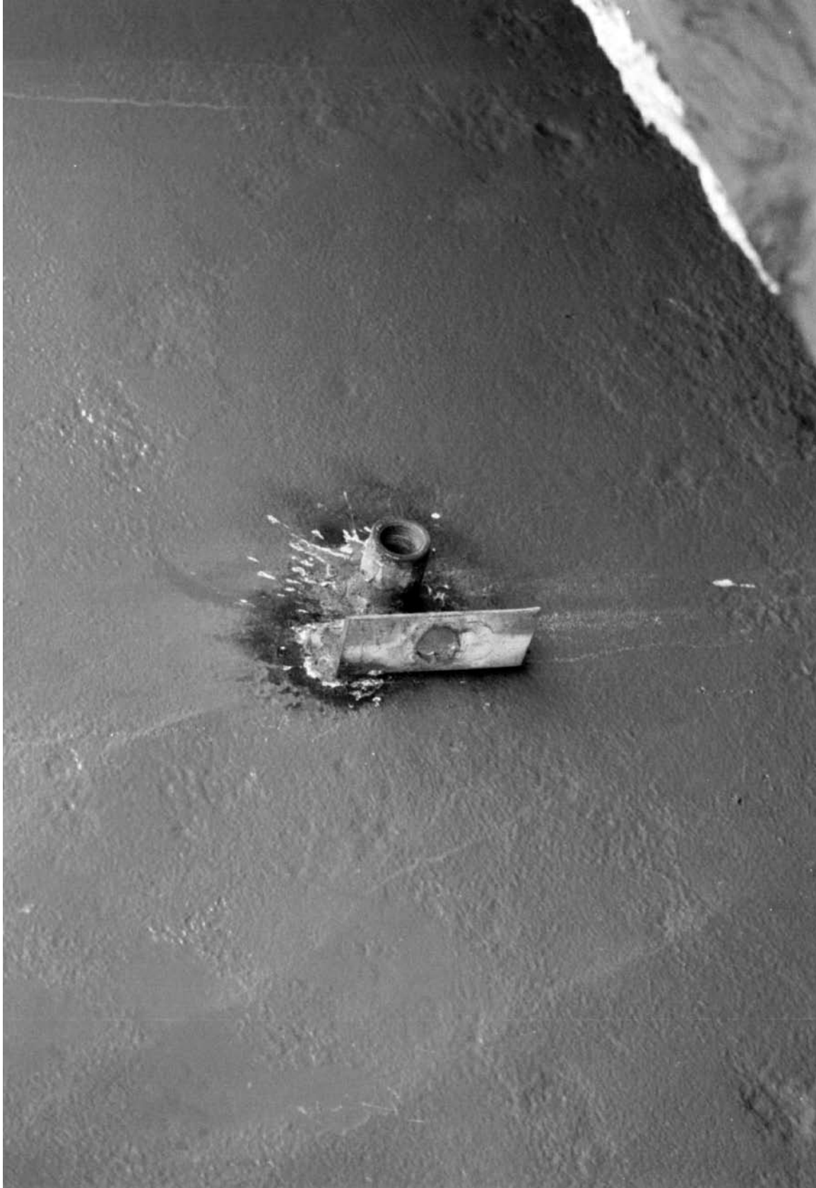
Closeup of hole used to insert CO 2 with coupling welded into place.
