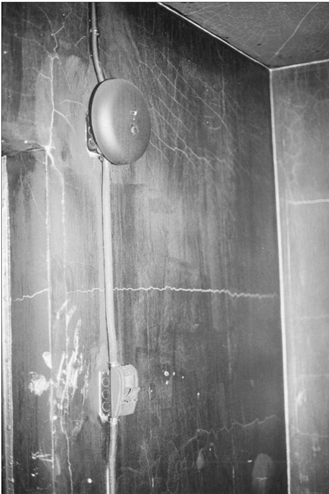
Manual fire alarm station and bell, third floor, at rear stair. Note extensive darkening soot.
