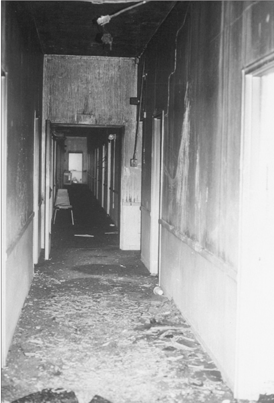
First floor corridor, looking to rear of building from lobby. Fire door in foreground was closed throughout much of the fire.
