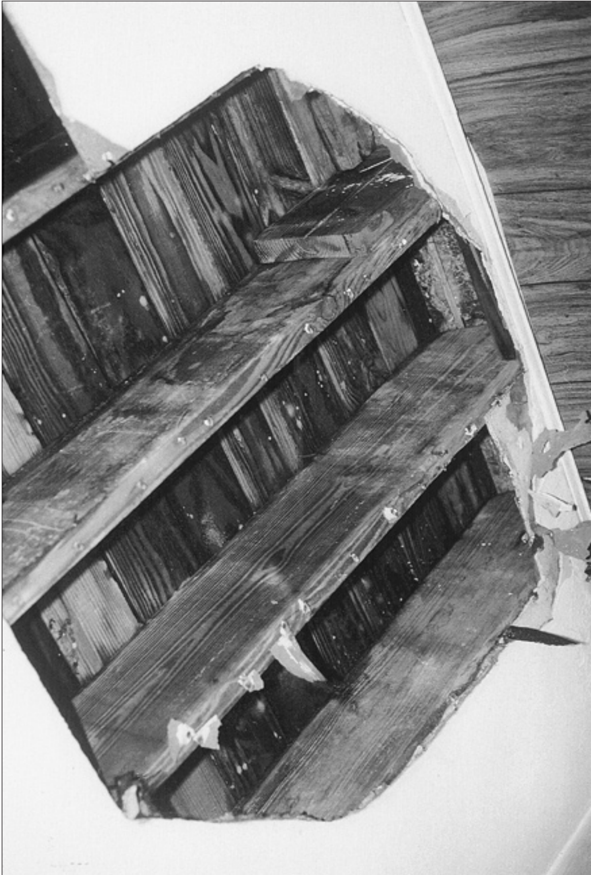
Typical floor construction, shown from ceiling of first floor room.
