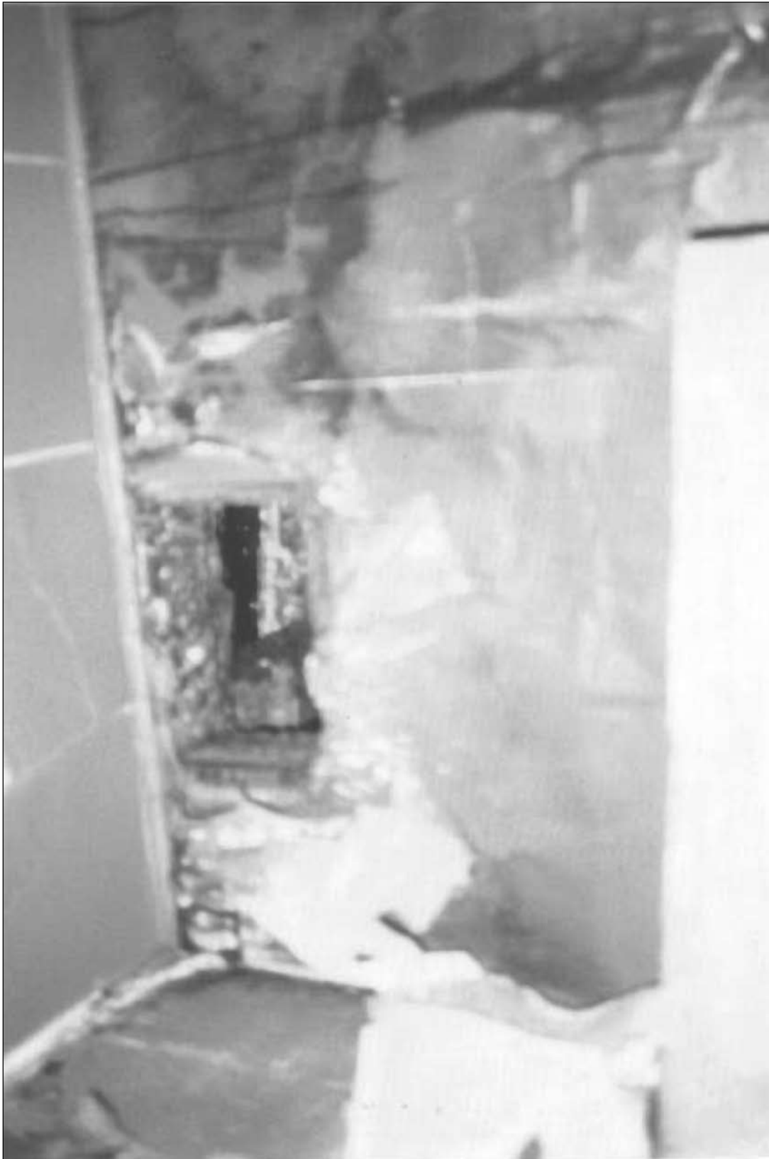
Photo by Randolph Kirby Smoke and heat traveled through air transfer vent from corridor to second floor south apartment in bedroom.
