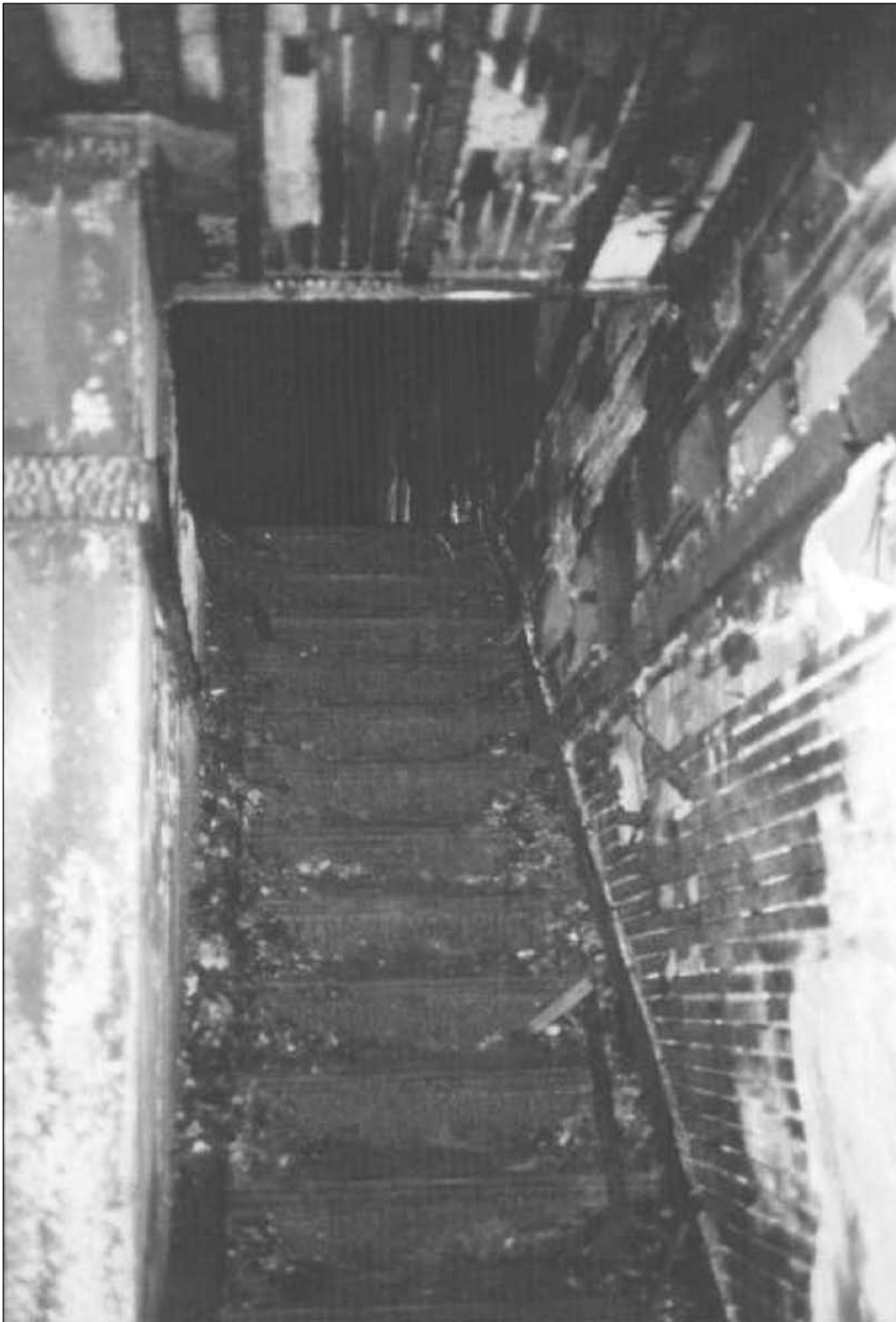
Stairway from first to second floor showing burn damage to staircase, wall, and ceiling.
