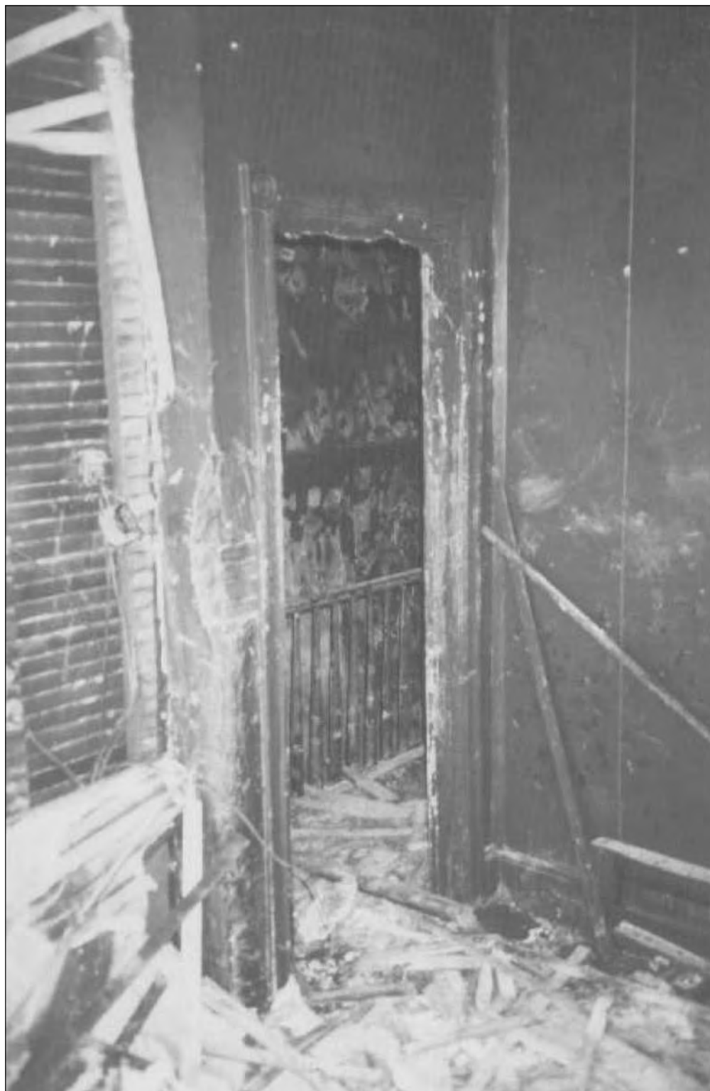
Entrance to second floor rear bedroom looking towards hallway. The door trim detail remains intact and heavy smoke residues stain the interior walls.
