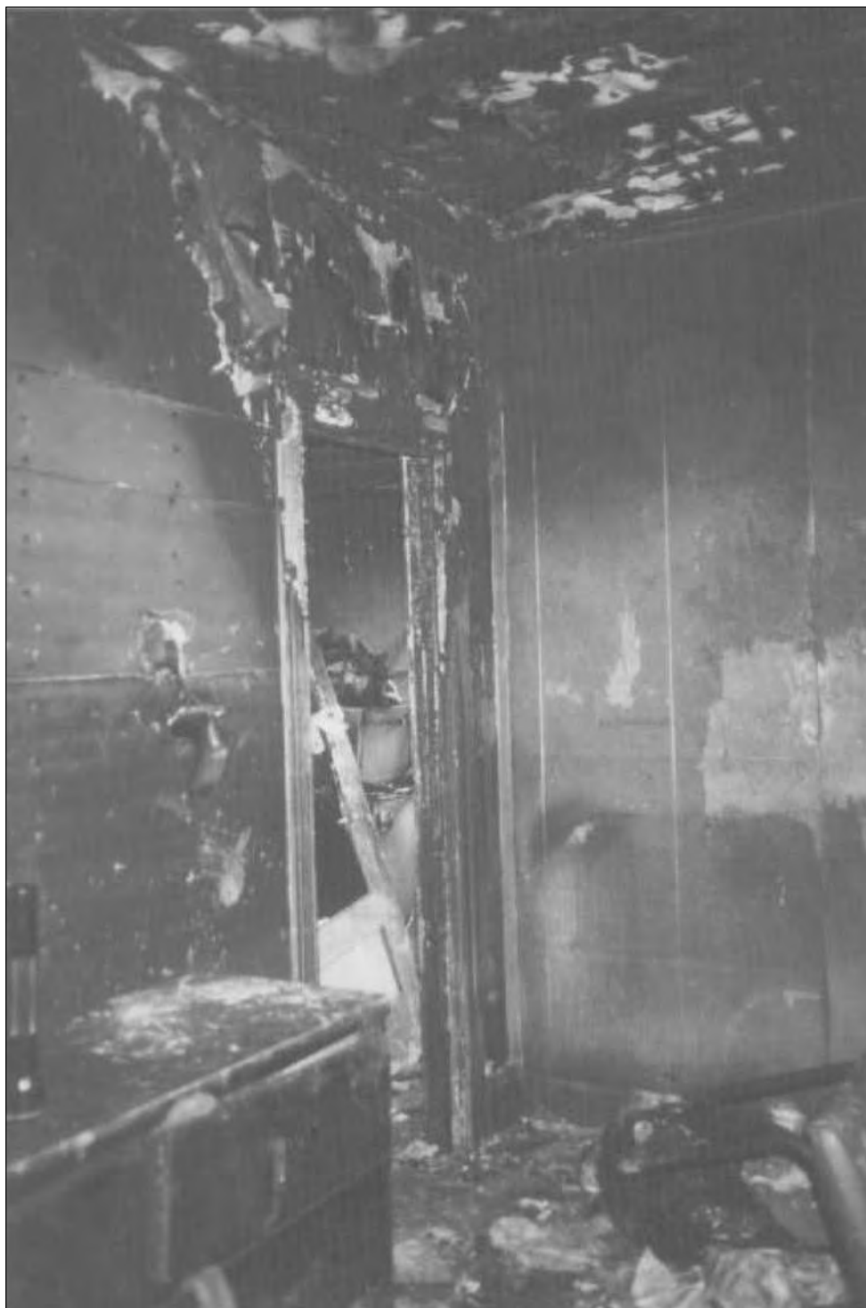
Thermal damage to wall and ceiling at top of front door opening to second floor center bedroom. This doorway was closed during the fire. However, convected heat and smoke from the fire below (see previous photograph) infiltrated the doorway through air gap at the top of the door.
