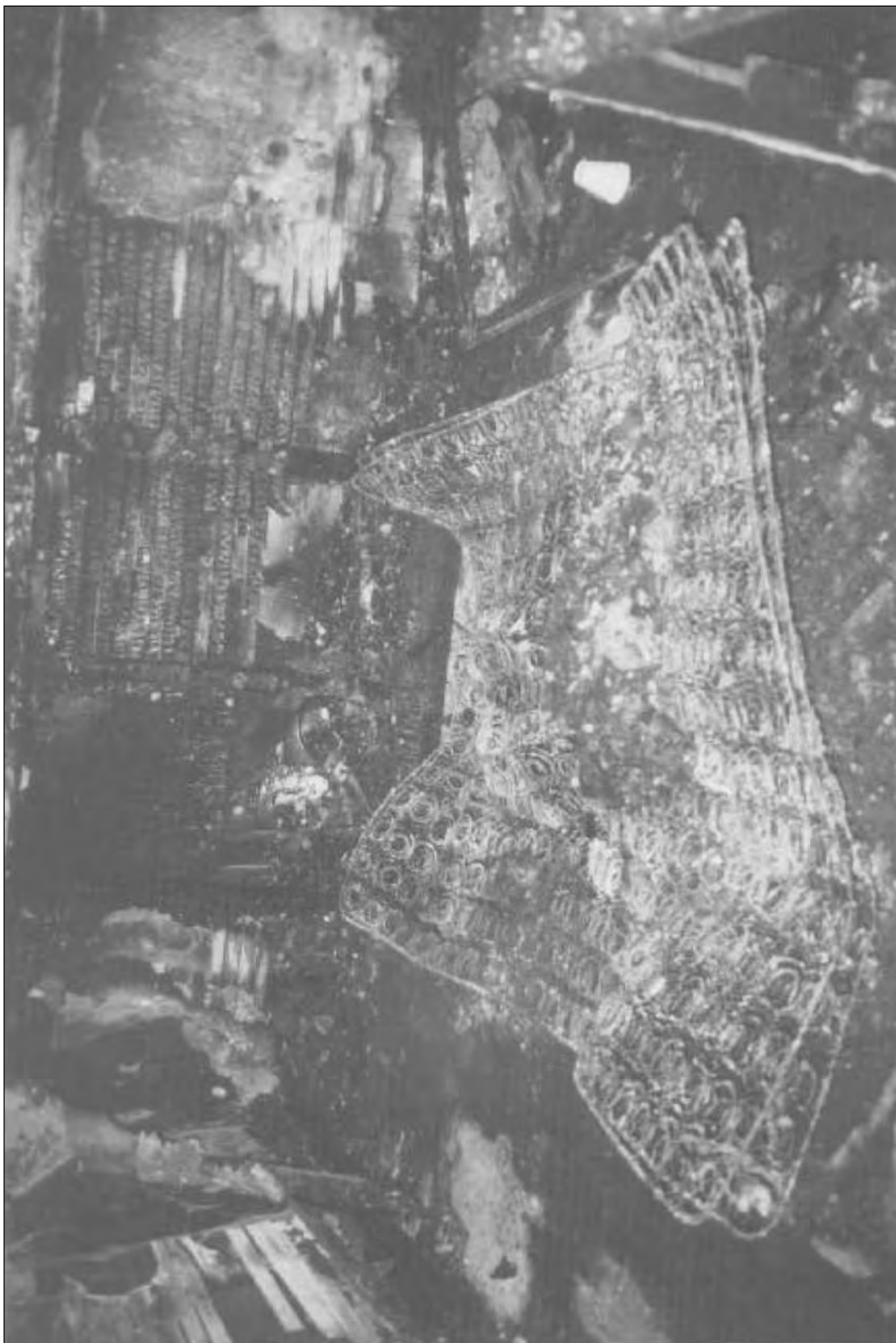
Point of origin in rear bedroom. The depressed floor area under the head of the bed was burned through to the crawl space below.
