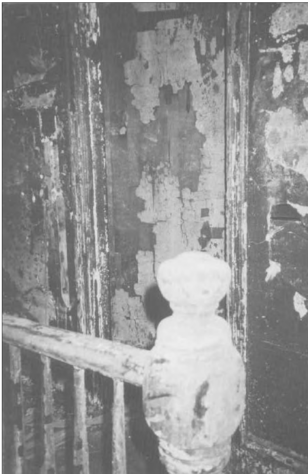
Rear doorway to second floor center bedroom. The homemade door is partially delaminated, explaining the irregular burn pattern.
