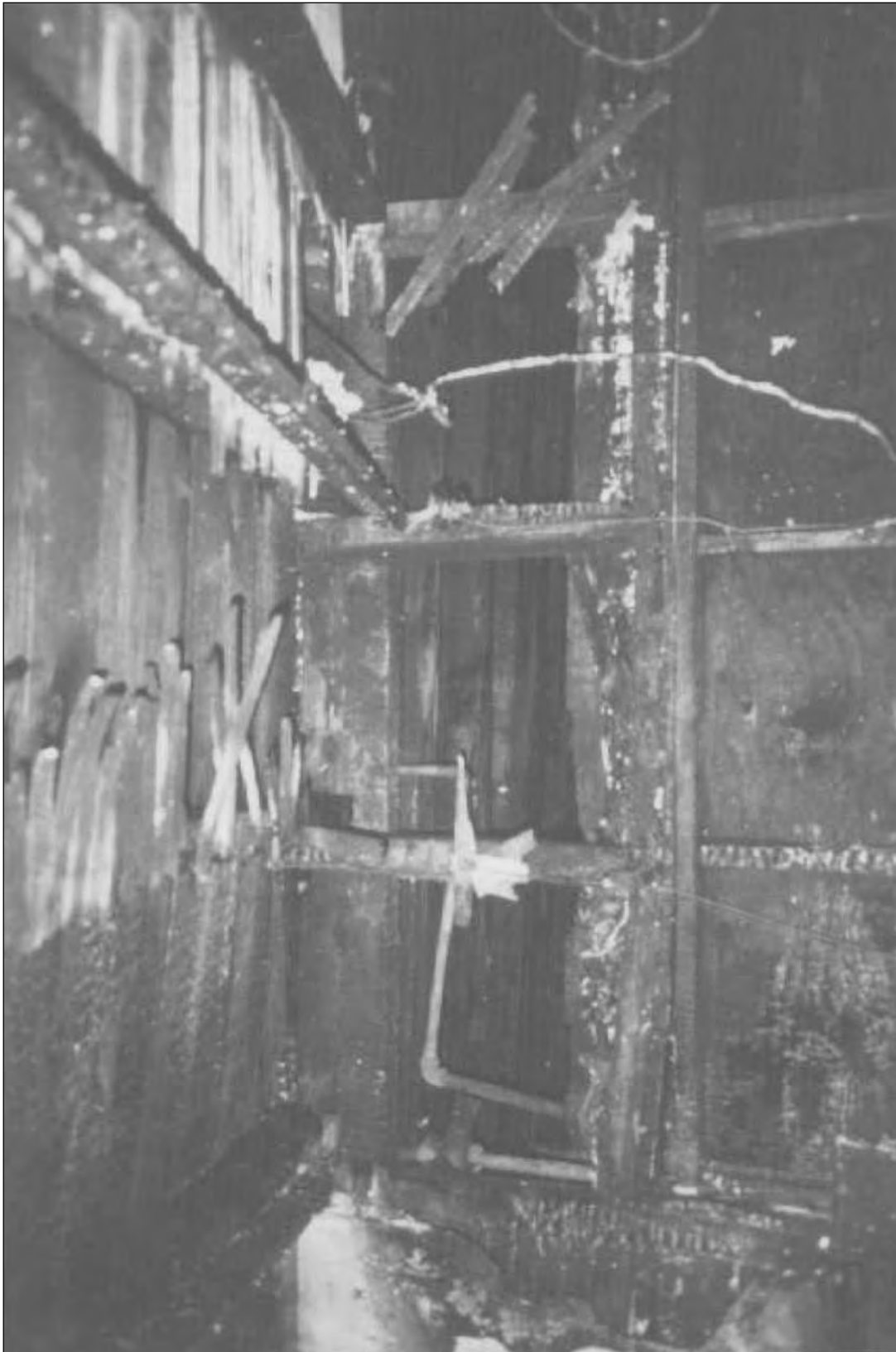
Wall and ceiling area above point of origin. Voids in the wall construction where the ceiling joists were attached permitted the fire spread horizontally into the kitchen and vertically into the rear exterior wall of the bedroom above.
