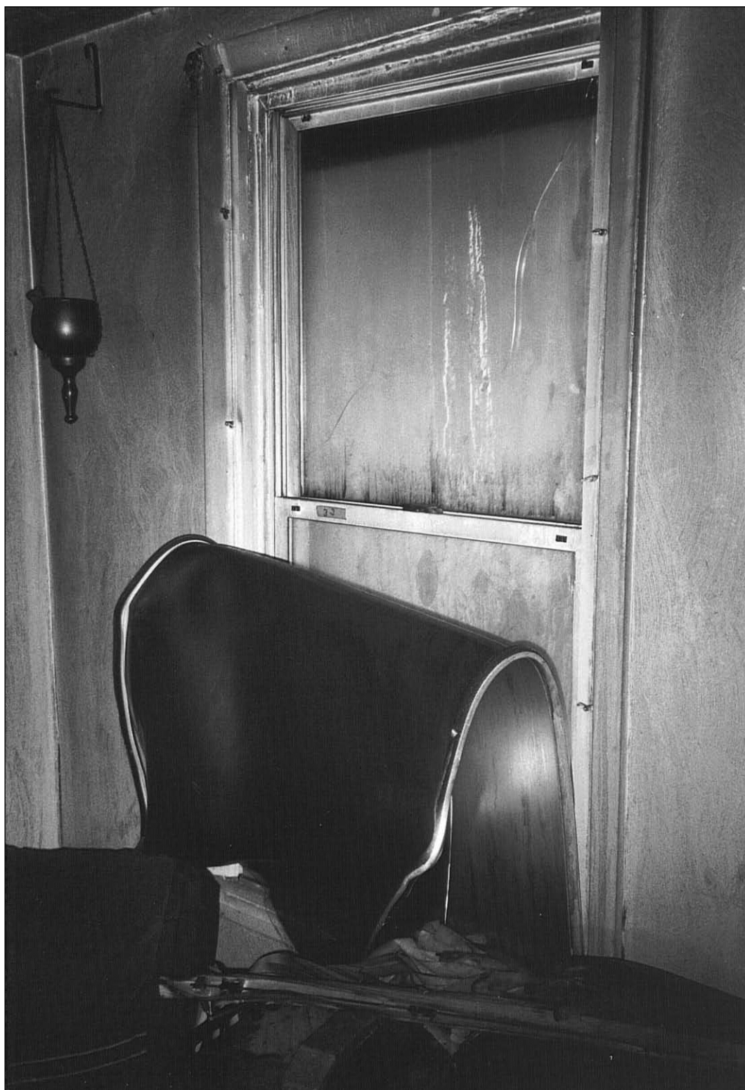
4. Window in corner of family room showing plastic panel which has partially melted and bent-over due to heat.
