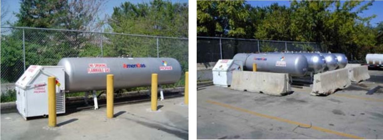
Figure 21. Original and upgraded LPG fueling station
