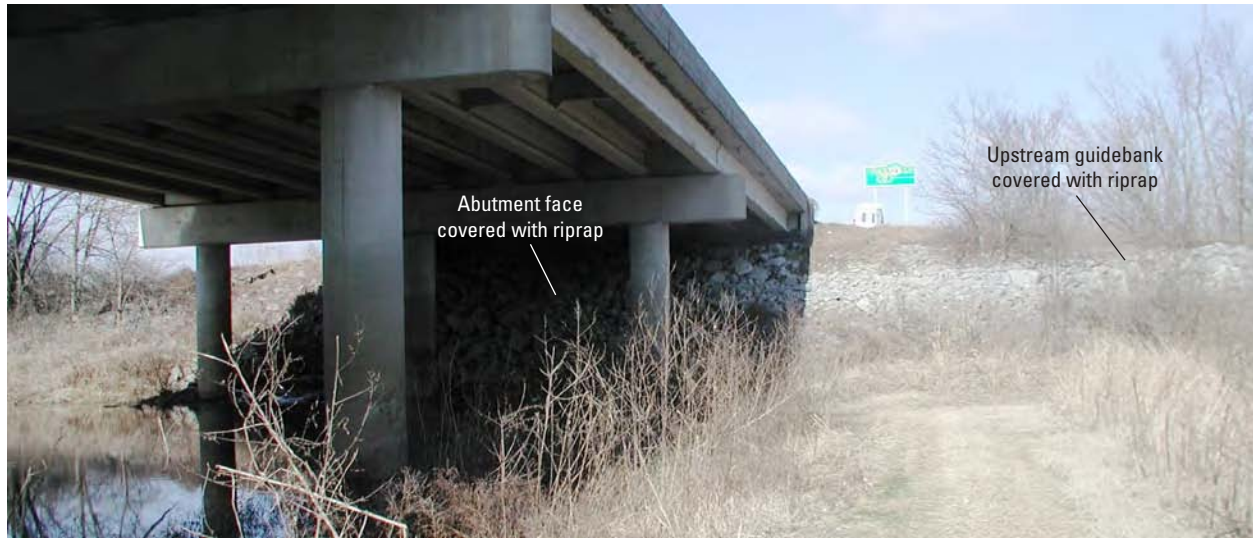
Figure 17. Abutment and part of the guidebank upstream from the right (northwest) end of structure A-1700 over the Mississippi River near Caruthersville, Missouri, January 23, 2007.
